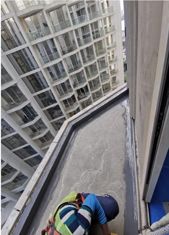
Waterproofing Works at Balcony Area Typical Floor
