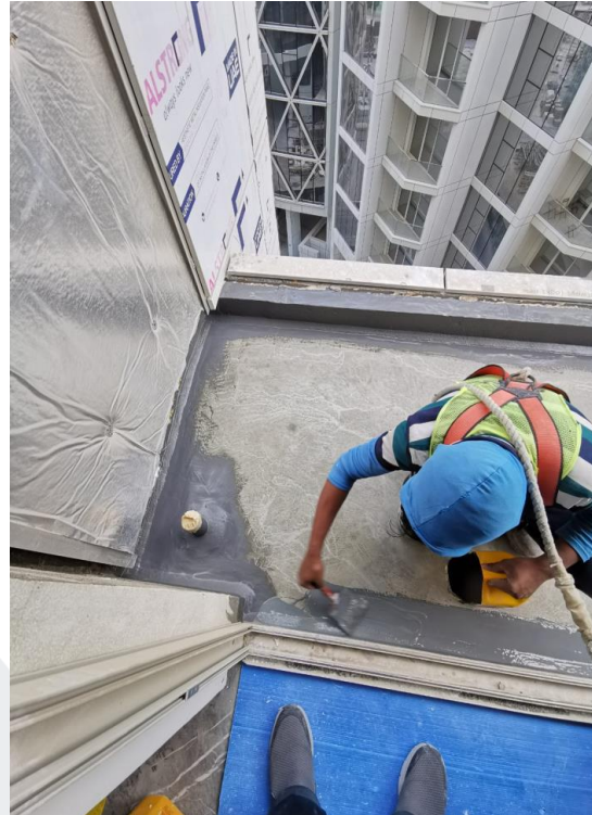
Waterproofing Works at Balcony Area Typical Floor
