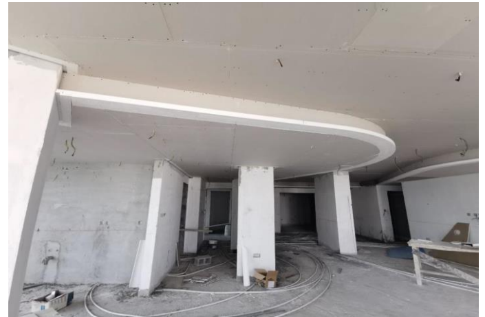
Gypsum Ceiling and Painting Works at Typical Floors
