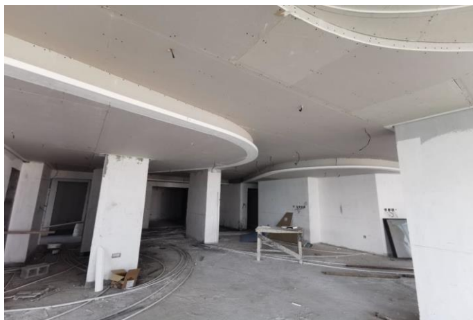
Gypsum Ceiling and Painting Works at Typical Floors
