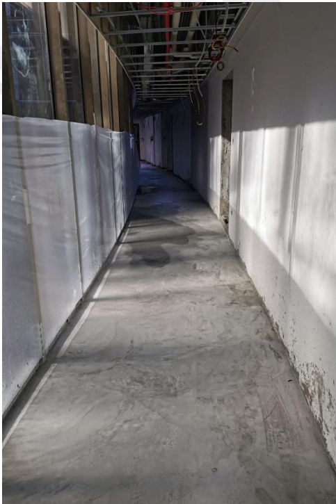
Screed Works for Corridor Area at Typical Floors
