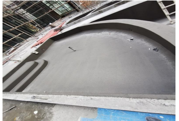
Application of Waterproofing for Swimming Pool Area at Ground Floor
