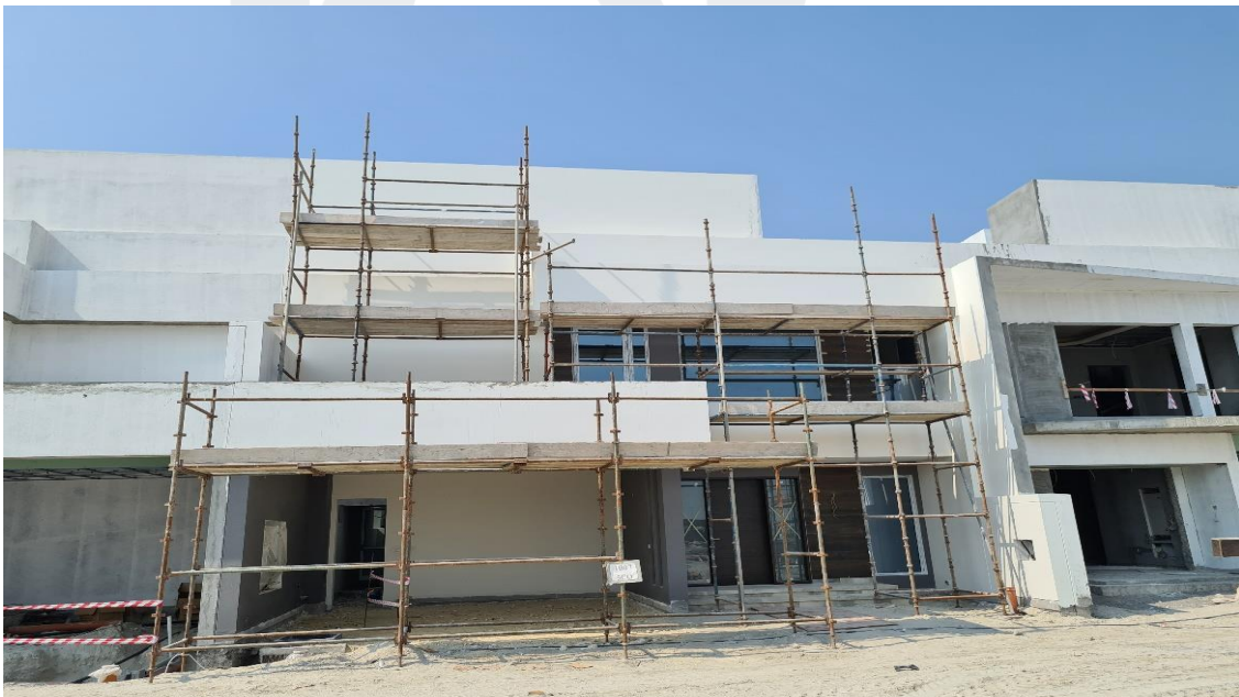
External Painting works in progress
