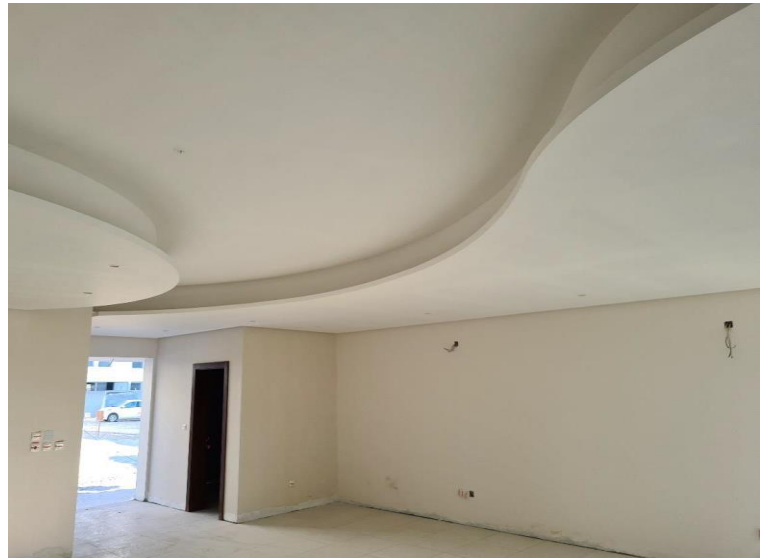
Internal Paint application in progress
