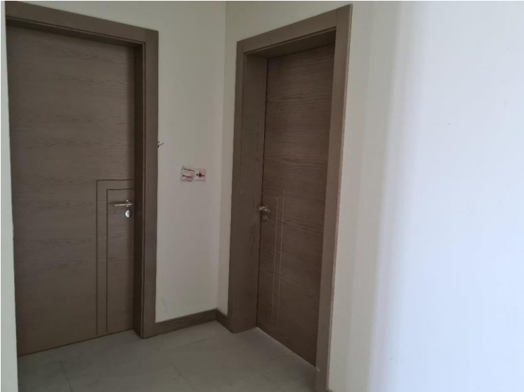
Wooden Doors & Skirting installation in progress
