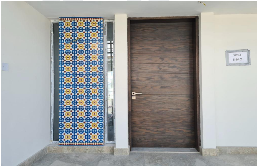
External Cladding Tile installation in progress
