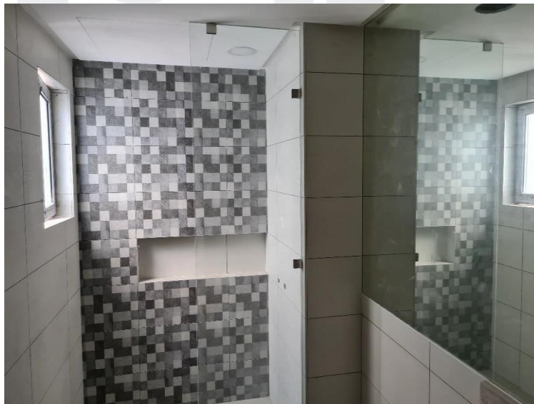
Toilet Shower Partition installation in progress
