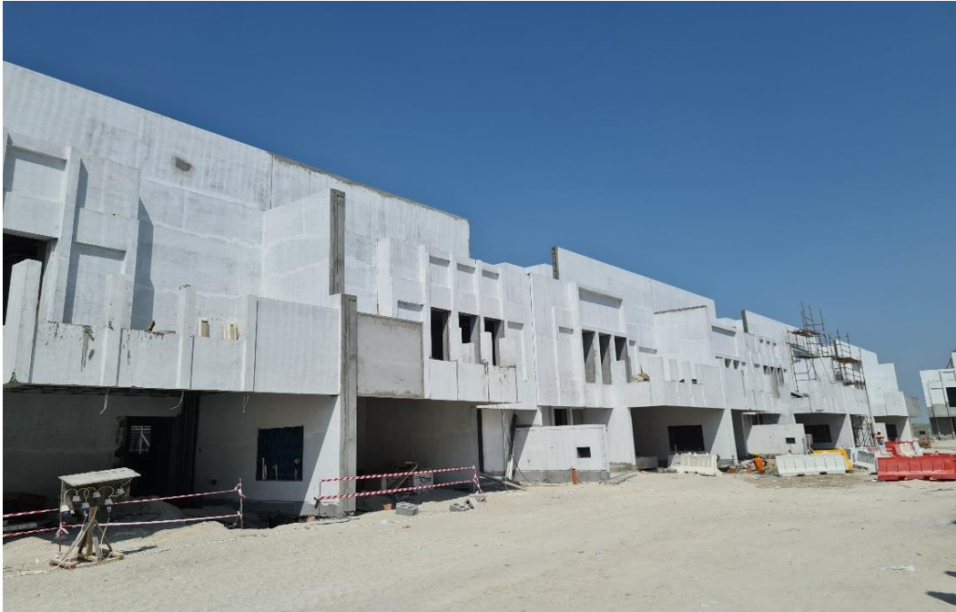
External Finishing works in progress
