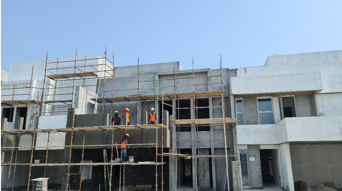
External Plastering preparation works in progress
