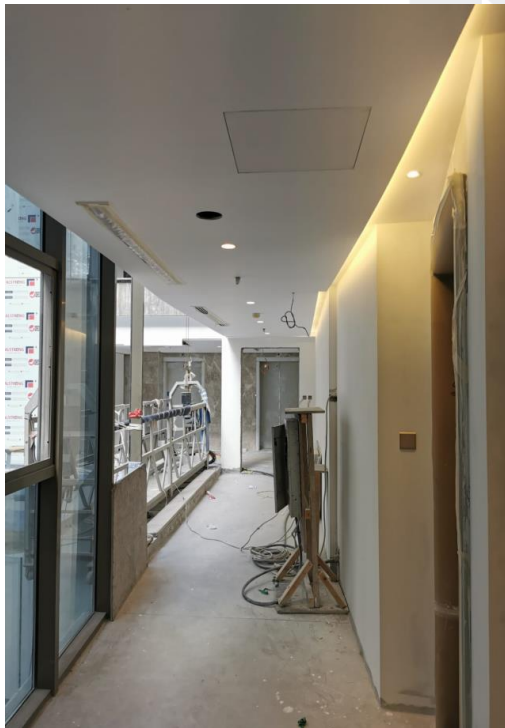
Gypsum Ceiling, Painting and Fixing of Lights for Corridor and Lift Lobby Area at Typical Floors
