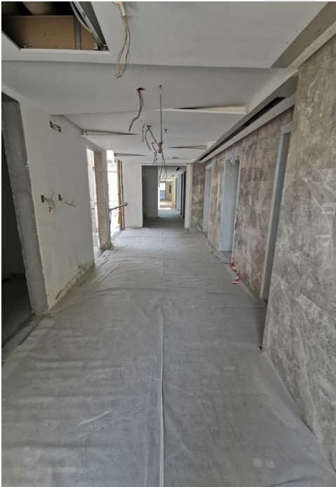
Gypsum Ceiling and Painting Works for Corridor Area at Typical Floors
