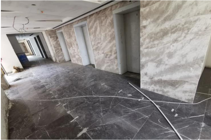
Gypsum Ceiling and Marble Wall Cladding Works for Lift Lobby Area at Typical Floors
