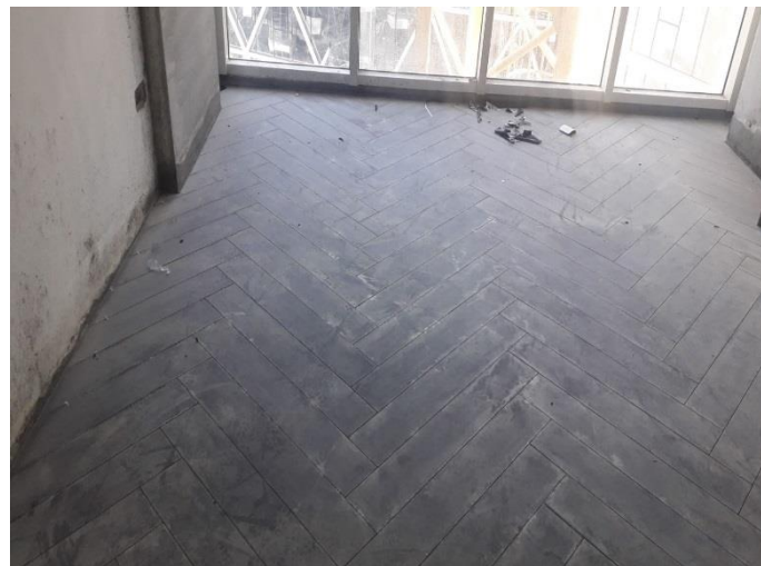
Tile Works at Typical Floors
