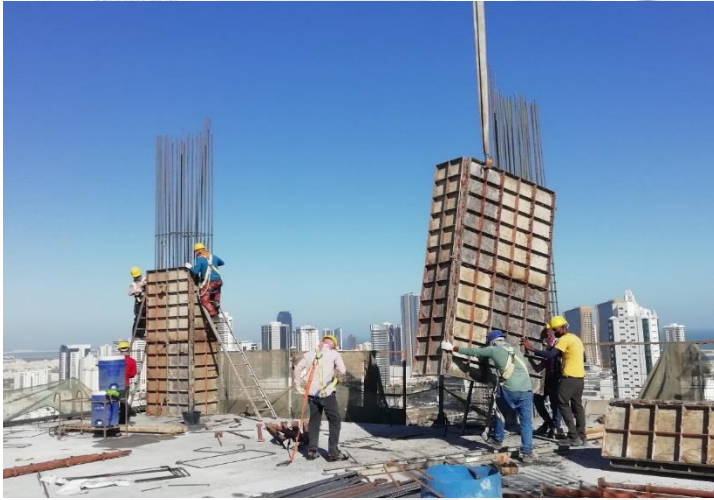
28 th Floor – Form Work for Column
