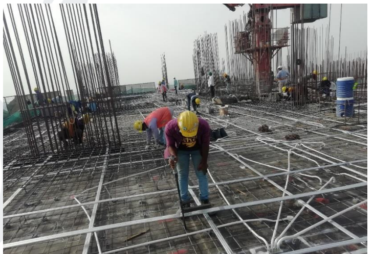
28 th Floor – Steel Work for Slab
