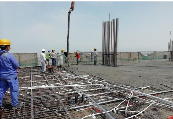
28 th Floor – Concrete for Slab
