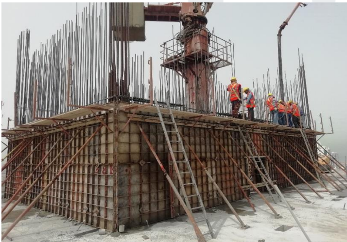
28 th Floor – Concrete Work for Shear Wall
