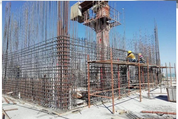
28 th Floor – Steel Work for Shear Wall
