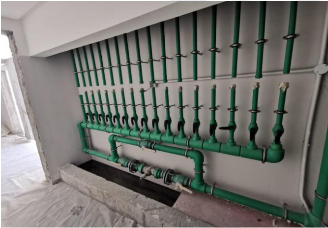
Installation of MEP Services at Typical Floors
