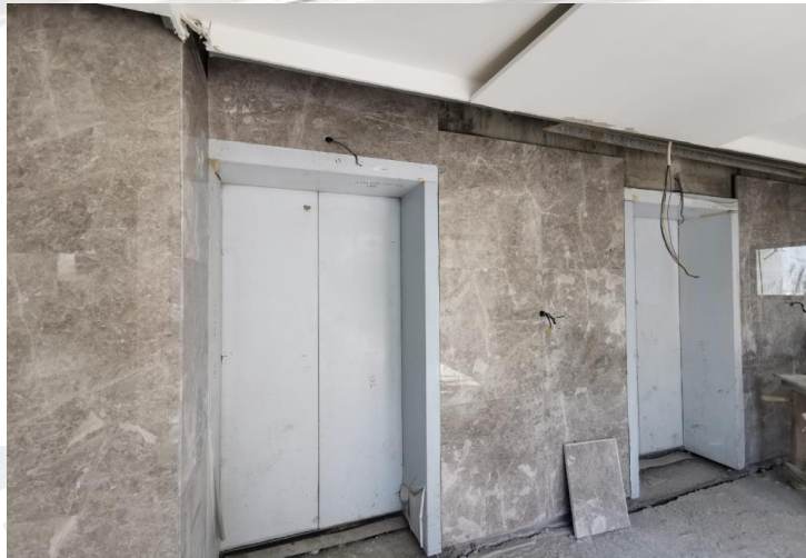
Marble Wall Cladding Work for Lift Lobby Area at Typical Floors
