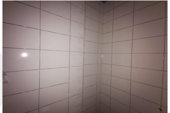
Tiling Works for Bathroom at Typical Floors
