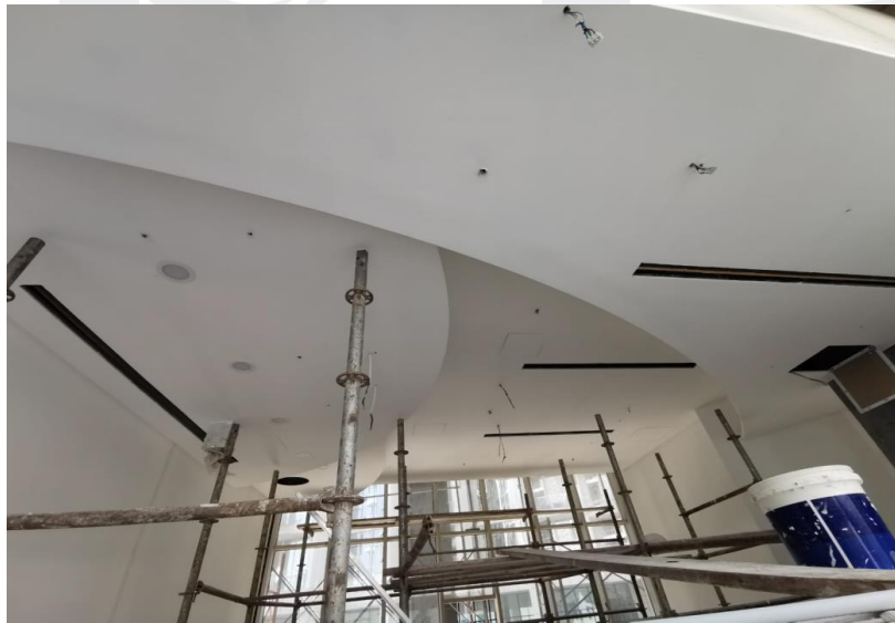
Gypsum Ceiling and Painting Works at Ground Floor
