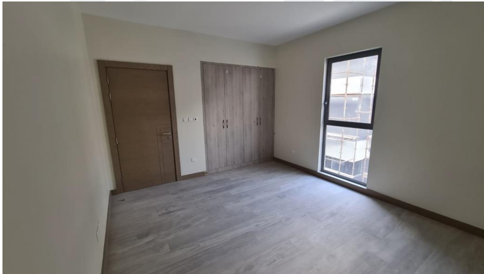
Floor Tile Works Final Finishing in Progress
