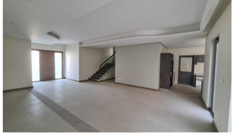
Internal Finishing Works in Progress
