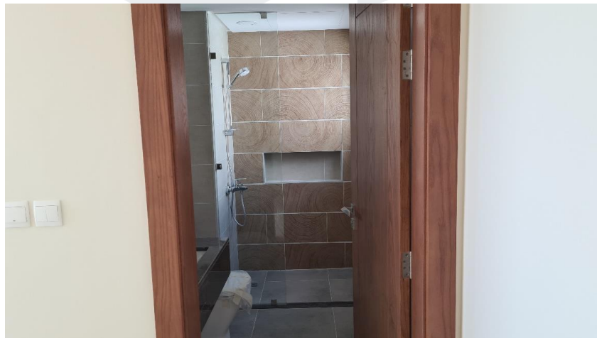
Villa Shower Partition Installation in Progress
