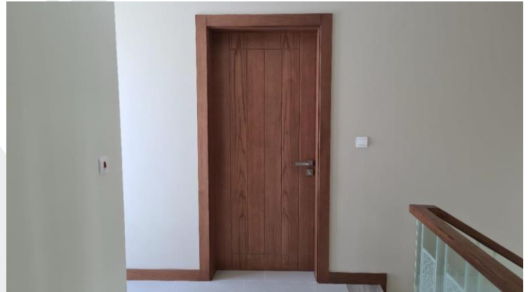
Internal Door Installation in Progress
