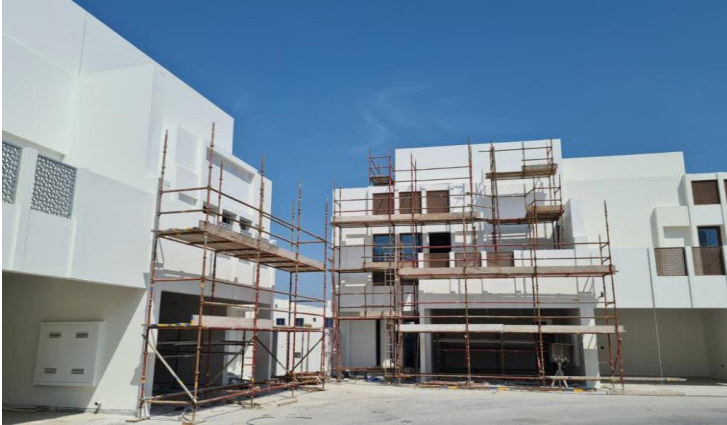
External Painting Works in Progress
