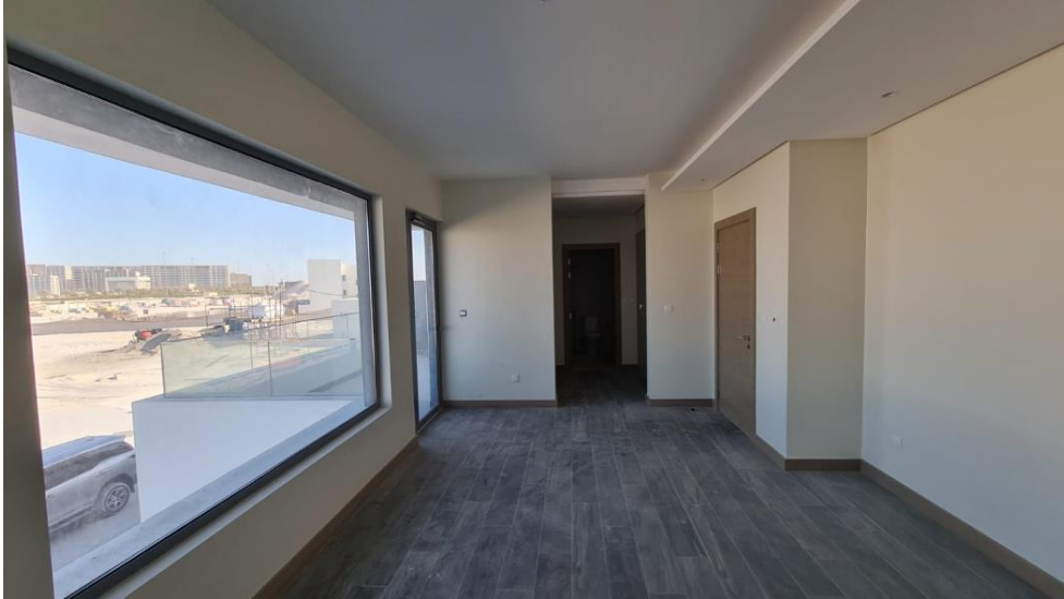
Internal Painting in Progress
