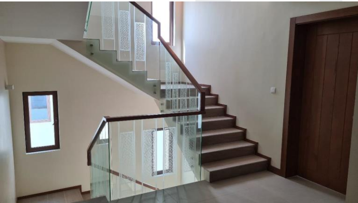
Staircase Handrail Installation in Progress
