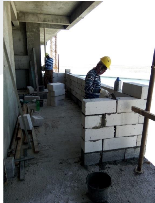
Zone 4 to 6 th Floor Block Works
