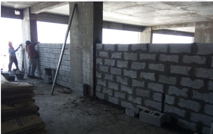
Zone 4 to 5 th Floor Block Works
