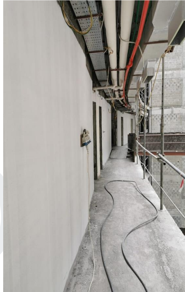
Plastering Works for walls at Typical Floors
