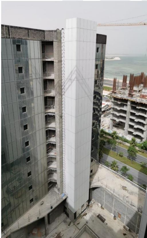
Installation of Aluminum Works (Brackets, Mullion, Rockwool, ACP Cladding and Glass and Application of Bitumen Paint)
