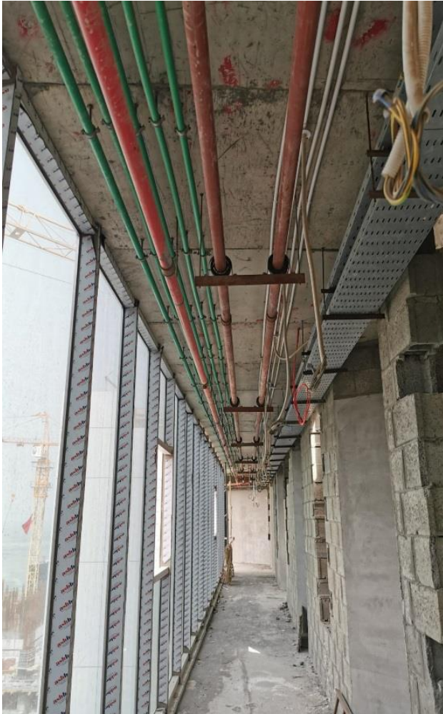
Installation of MEP Services at Typical Floors
