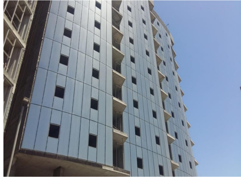
Installation of Aluminum Works (Brackets, Mullion, Rockwool, ACP Cladding and Glass and Application of Bitumen Paint)
