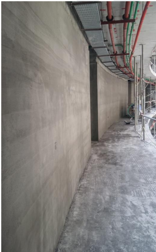
Plastering Works for Walls at Typical Floors
