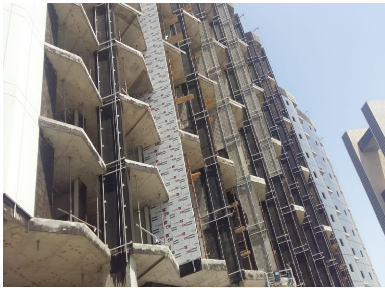
Installation of Aluminum Works (Brackets, Mullion, Rockwool, ACP Cladding and Glass and Application of Bitumen Paint)
