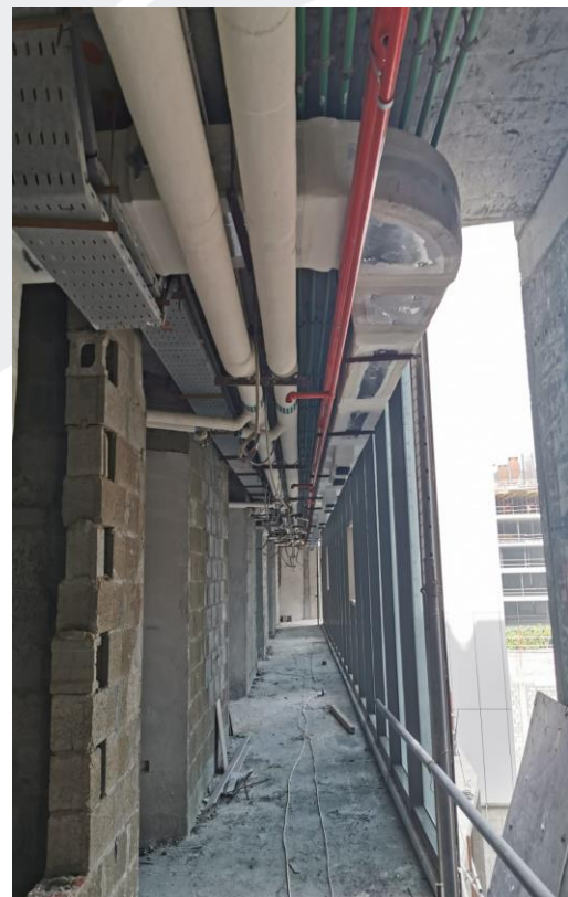
Installation of MEP Services at Typical Floors
