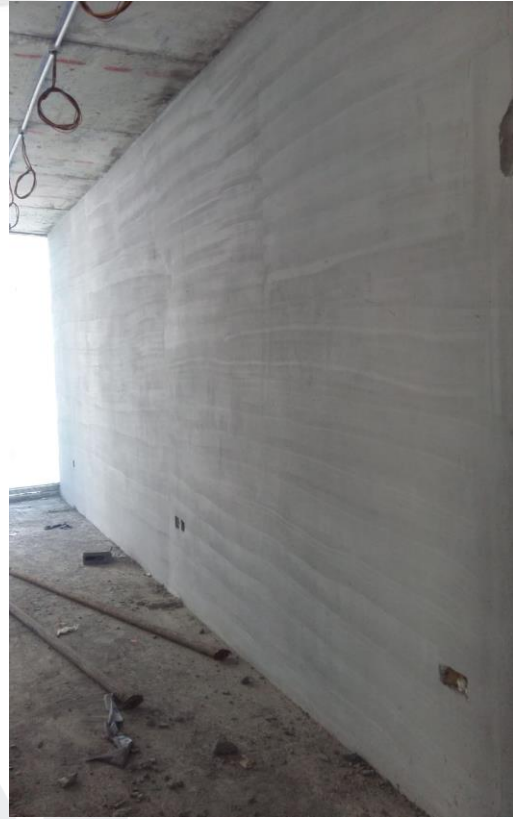
Plastering Works for Walls at Typical Floors
