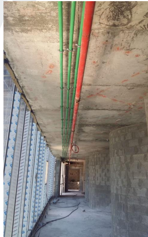
Installation of MEP Services at Typical Floors
