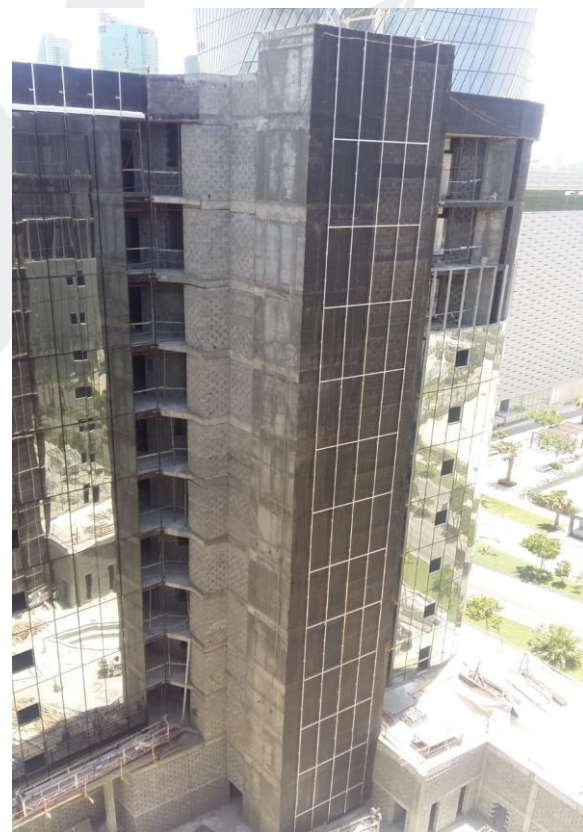
Installation of Aluminum Works (Brackets, Mullion, Rockwool, ACP Cladding and Glass and Application of Bitumen Paint)
