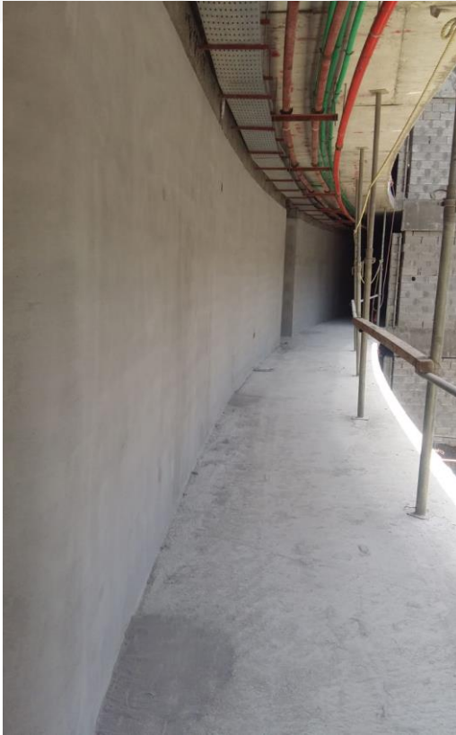
Plastering Works for Walls at Typical Floors
