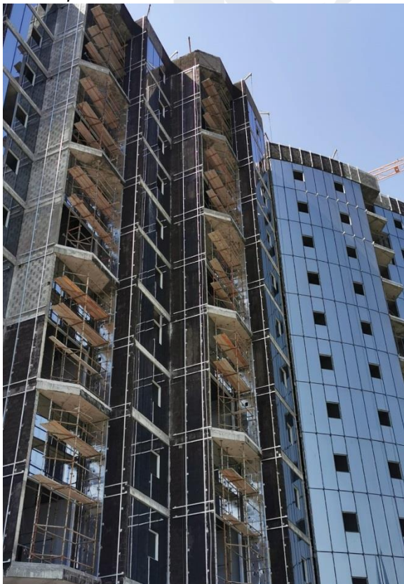
Installation of Aluminum Works (Brackets, Mullion, Rockwool, ACP Cladding and Glass and Application of Bitumen Paint)
