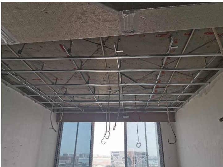
Ceiling Framing Works at Typical Floors
