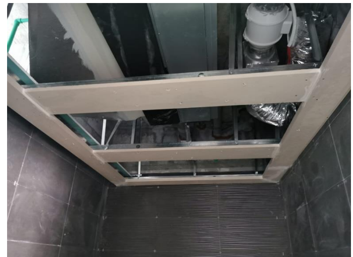
Ceiling Framing and MEP Services Works at Typical Floors
