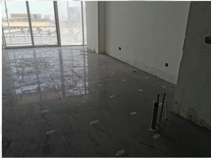
Marble Works for Rooms at Typical Floors
