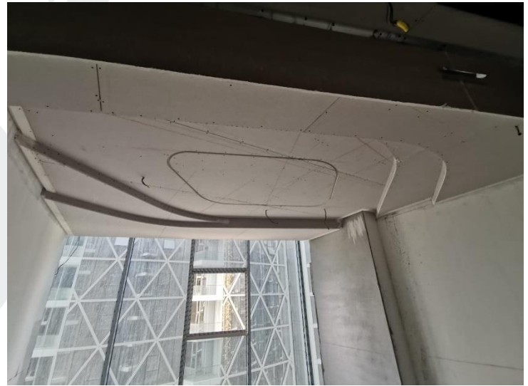
Ceiling Works at Typical Floors
