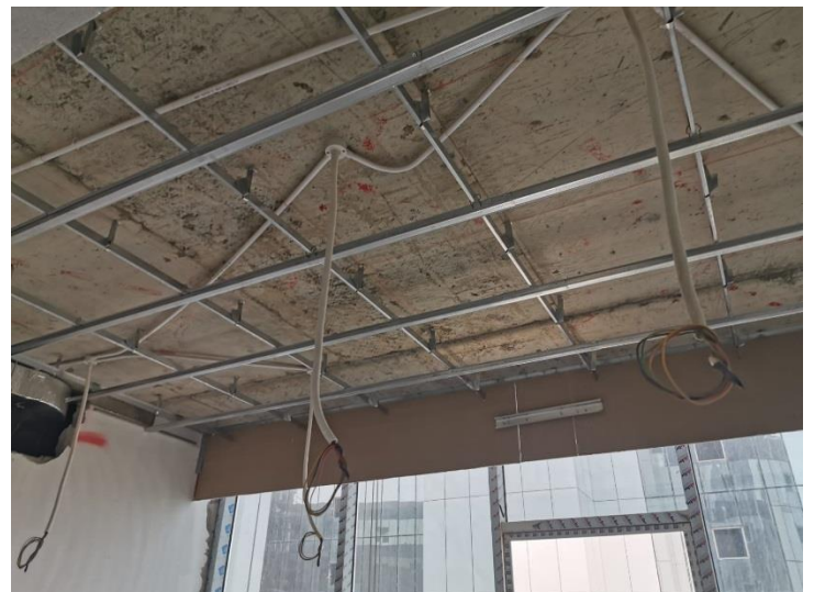
Ceiling Framing Works at Typical Floors
