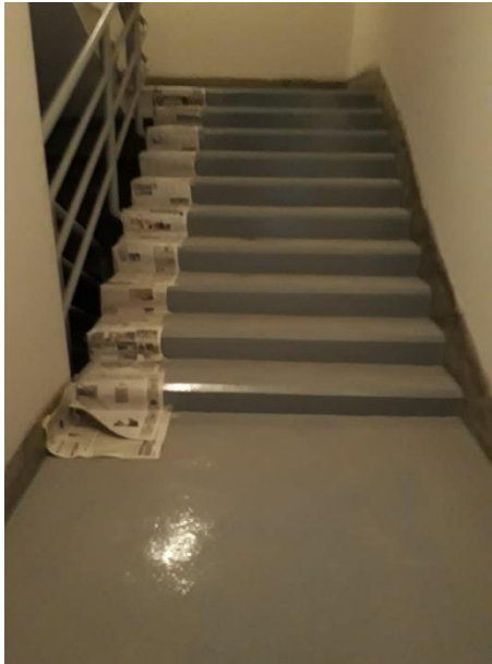
Staircase Epoxy Handrail
