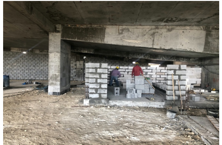
Ground Floor Block Works
