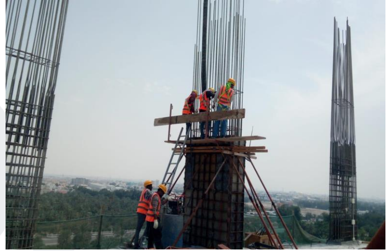
9 th Floor – Column Concrete
