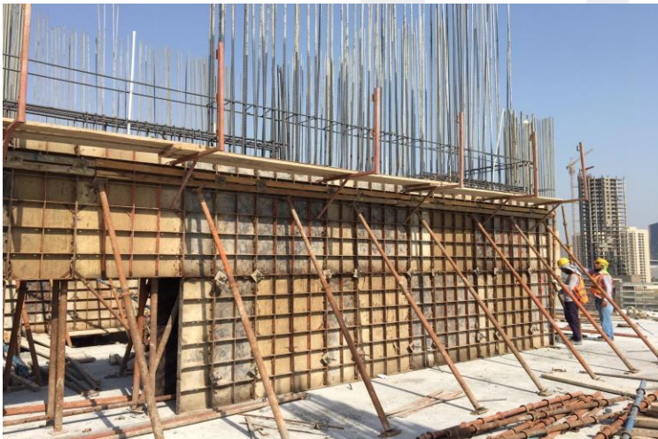
9 th Floor – Shear Wall Shuttering
