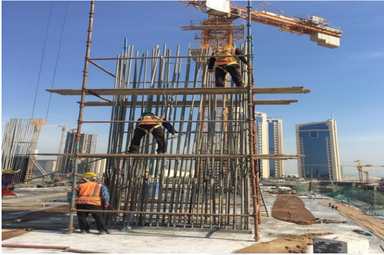
9 th Floor – Column Steel Works
