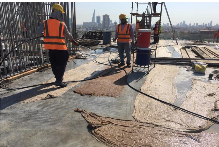
9 th Floor Slab – Curing Work
