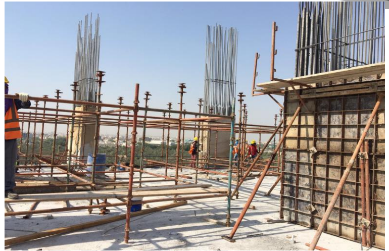
9 th Floor – Shuttering Work
