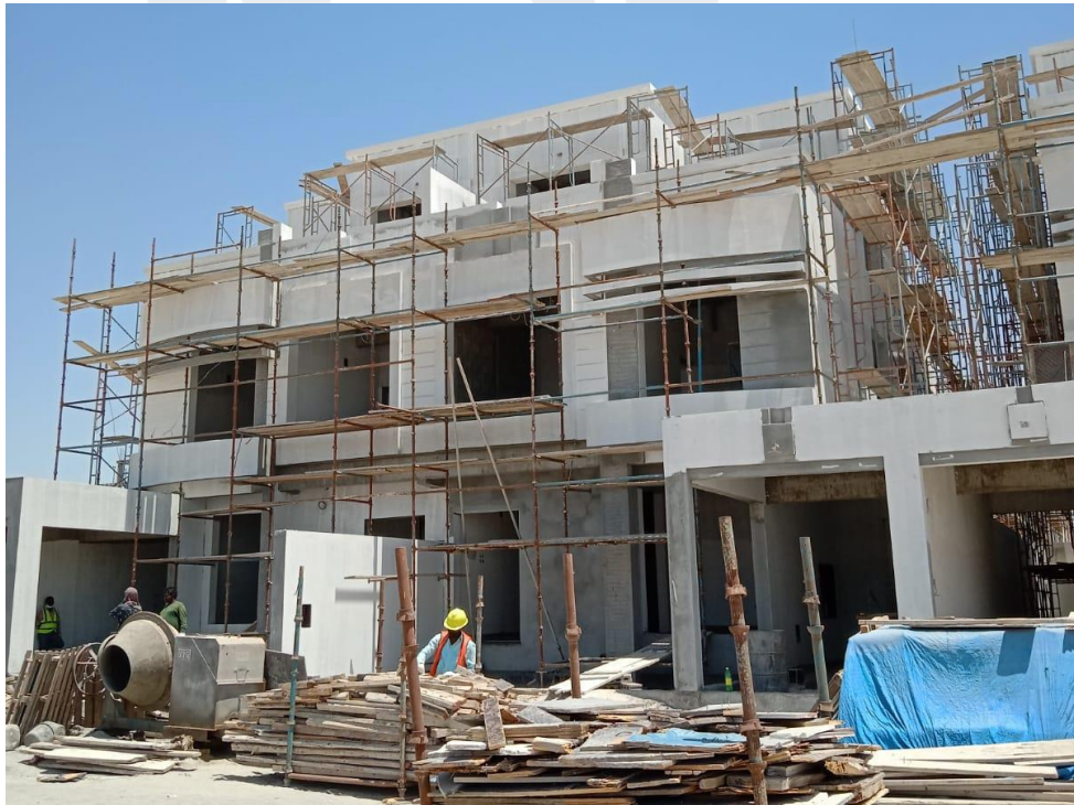
Villa 5 & 6 Overall View
