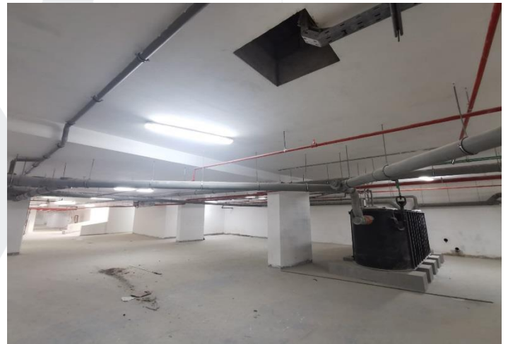
Basement 1 Painting Works
