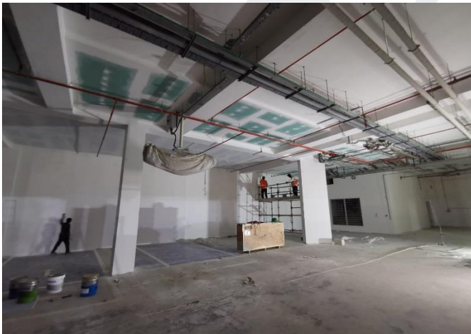
Basement 2 Light Fixing
