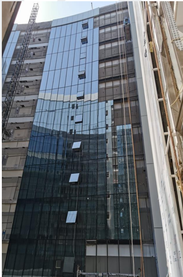
Glazing Work Front Portion
