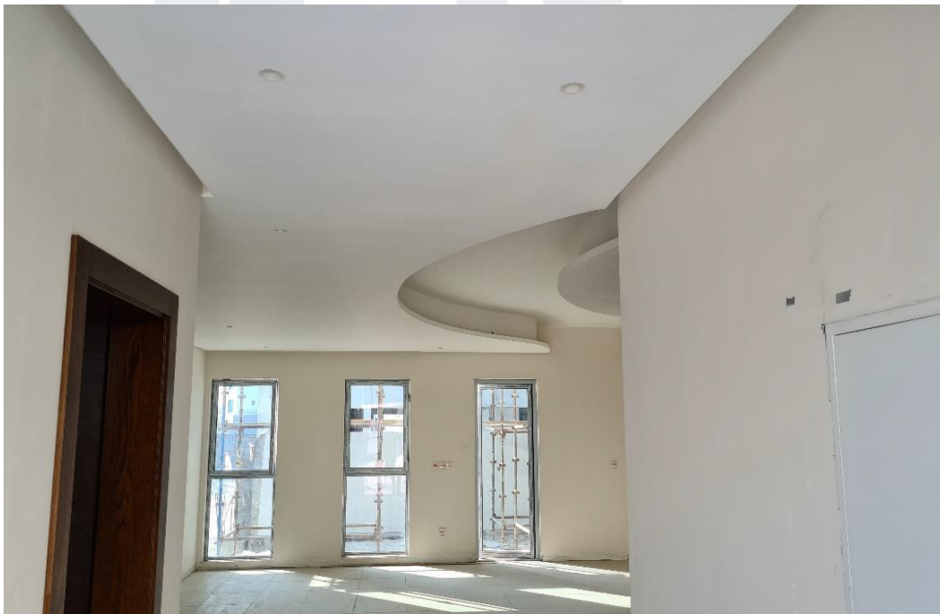
Villas Ceiling works in progress
