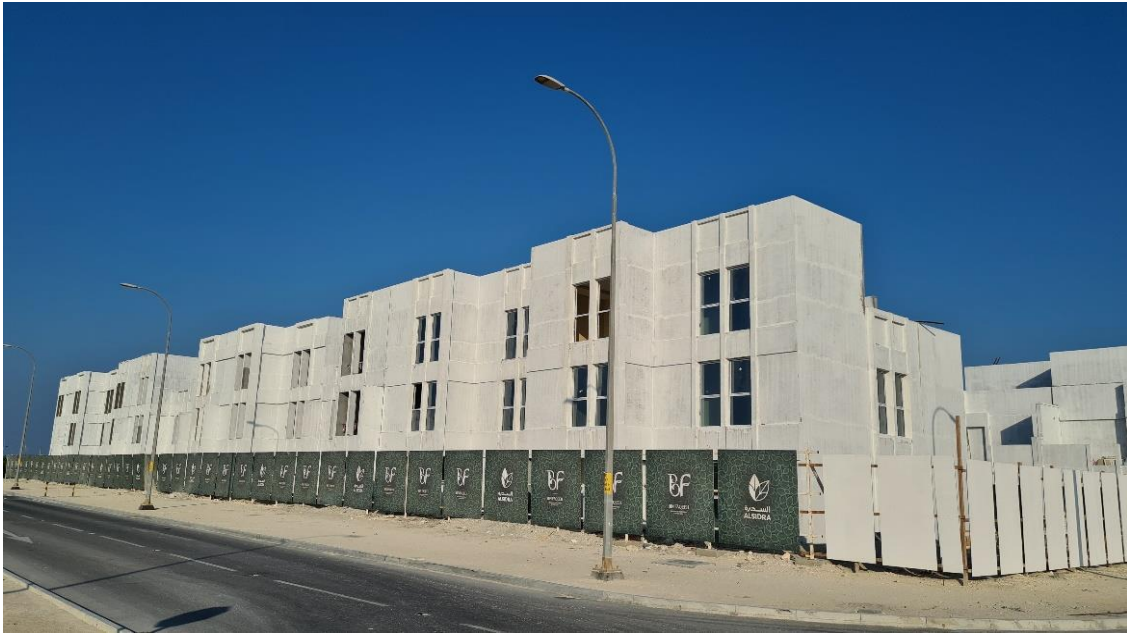
External Street View
