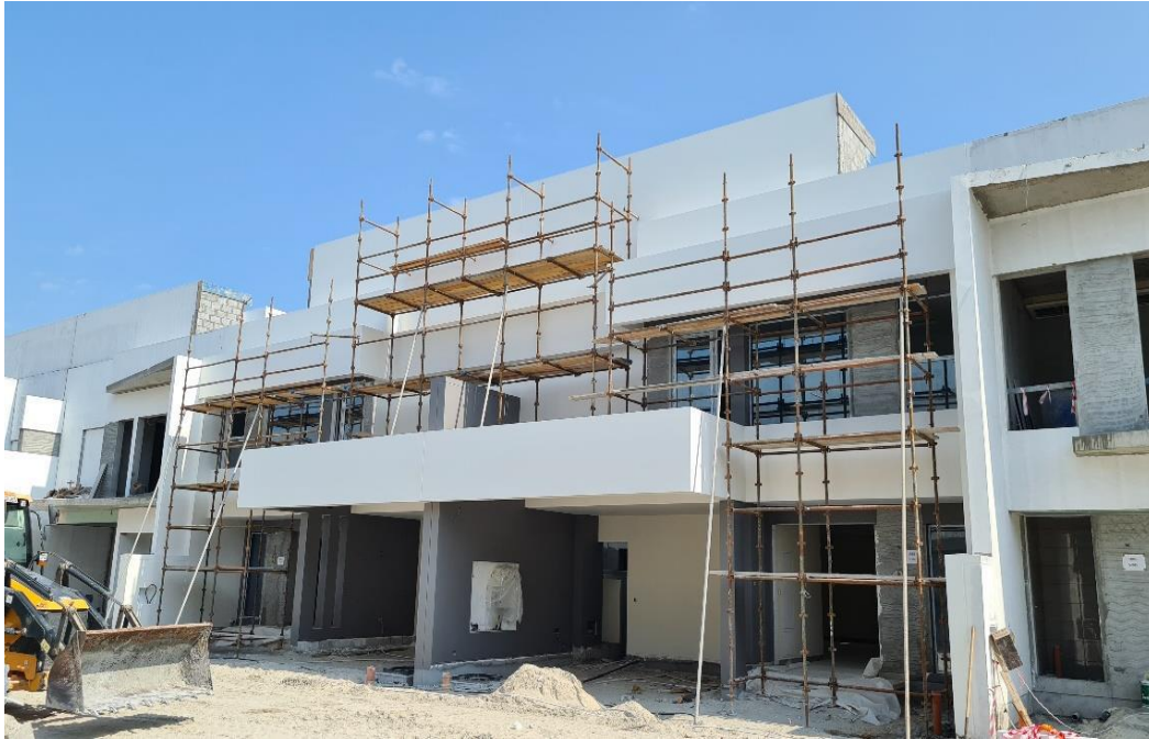
External Cladding Tile Installation in progress
