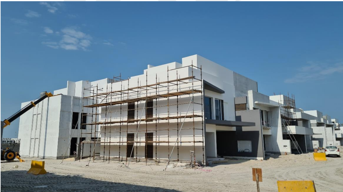
External Painting works in progress
