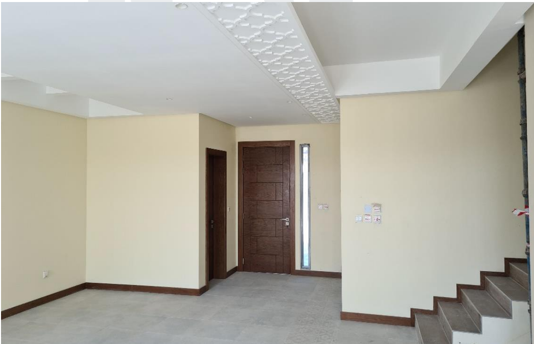
Internal Paint application in progress
