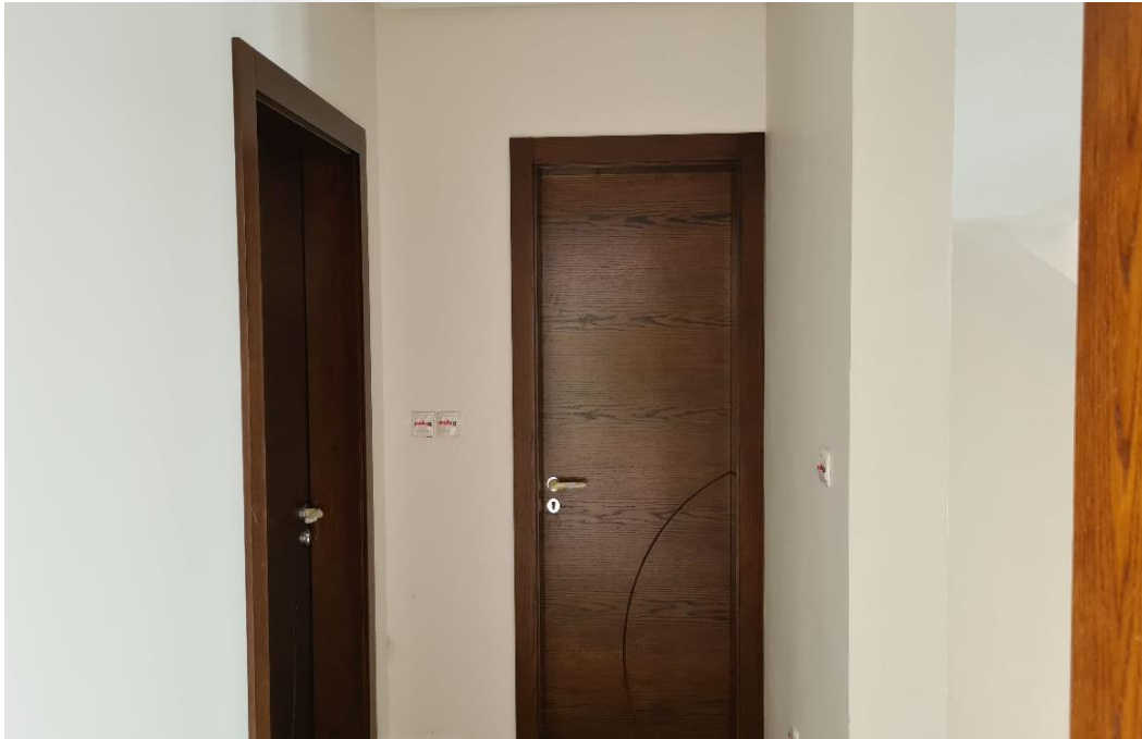
Wooden Doors & Skirting installation in progress
