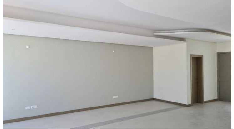
Internal Finishing Works in Progress
