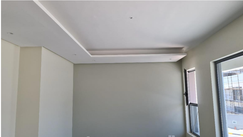
Internal Painting in Progress
