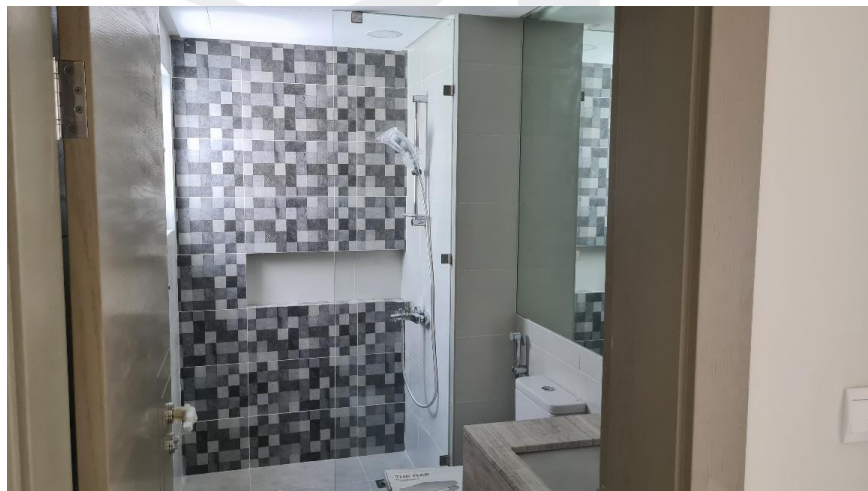
Staircase Handrail installation in progress
