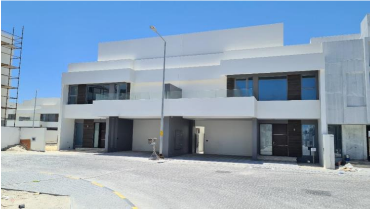
External Painting Works in Progress
