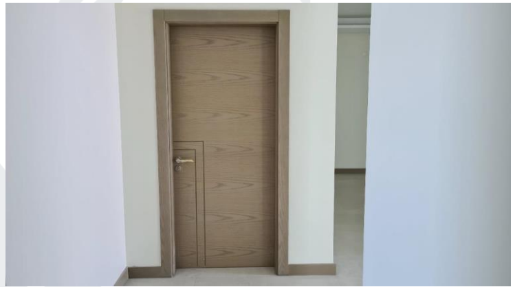
Internal Door Installation in Progress
