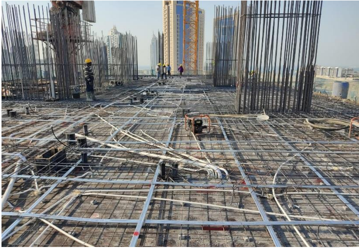
17 th Floor Slab Reinforcement Work
