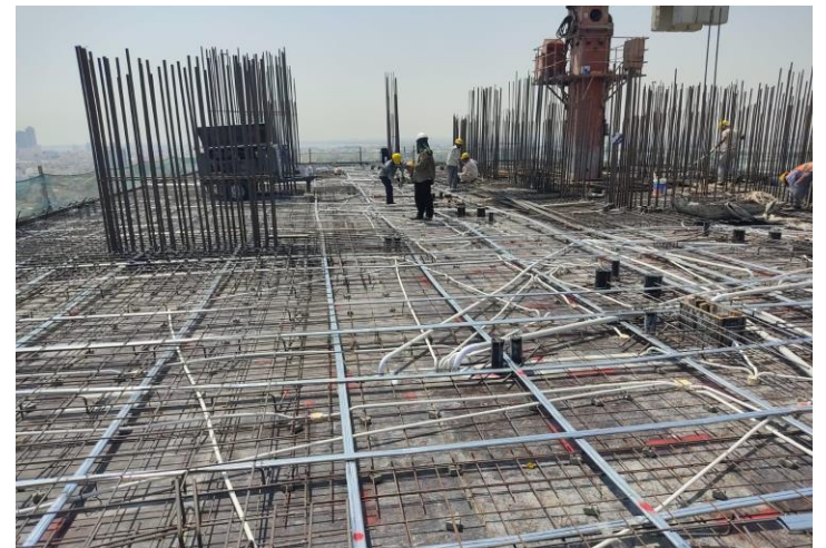
15 th Floor – Slab Reinforcement Work
