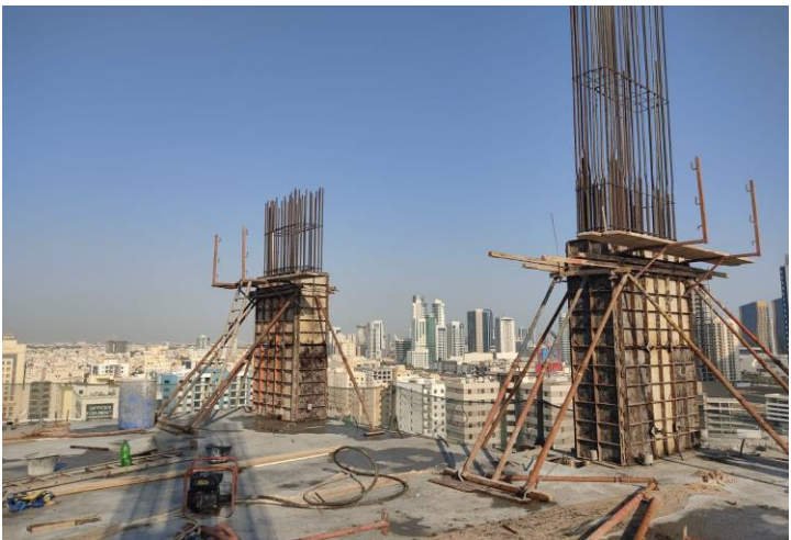
14 th Floor – Column Shuttering Work
