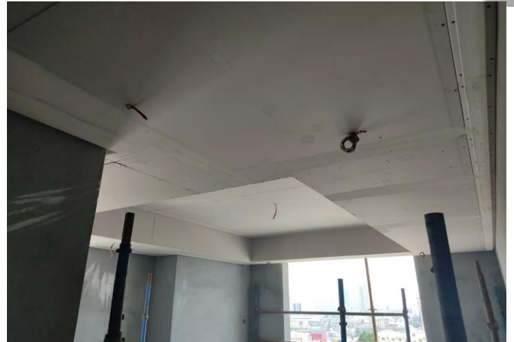
8 th Floor Gypsum Ceiling Work
