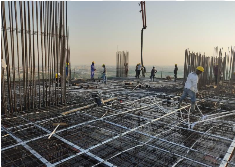
15 th Floor Slab Concrete Works
