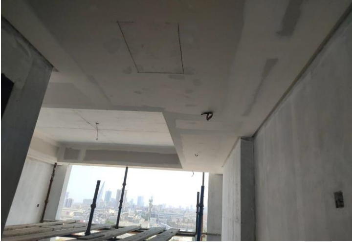
8 th Floor Gypsum Ceiling Work
