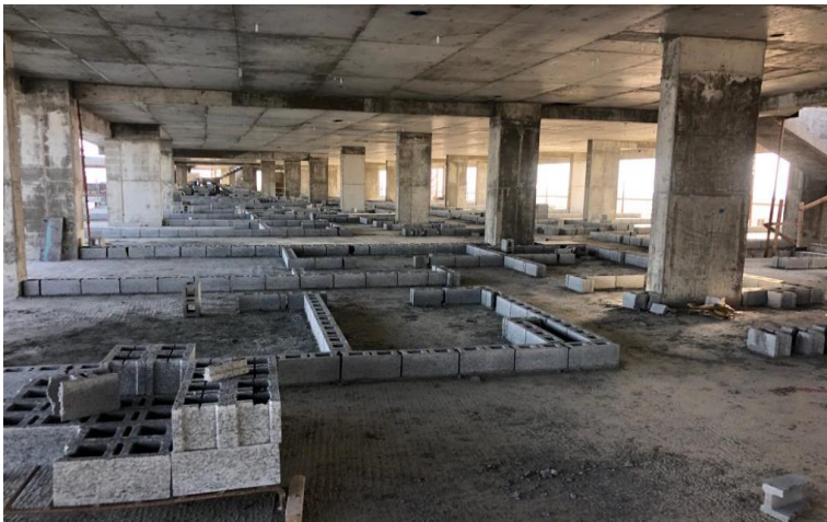
Zone 5 – 6 th Floor Block Work Setting Out
