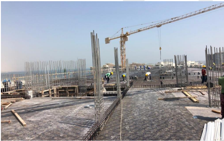
Zone 2 – 6 th Floor Slab & Beam Shuttering and reinforcement, Slab Concrete Works
