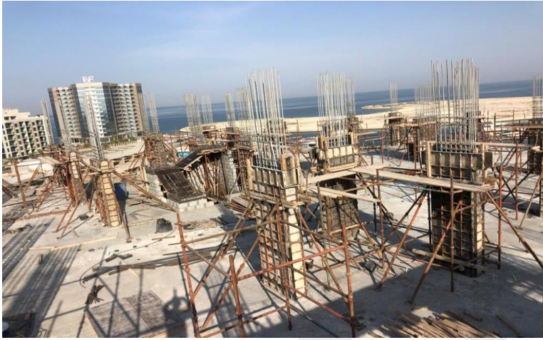
Zone 1 – 5 th Floor Column and Wall Shuttering Work
