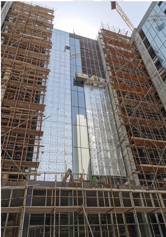
Installation of Aluminum Works (Brackets, Mullion, Rockwool ACP Cladding & Glass and Application of Bitumen Paint)
