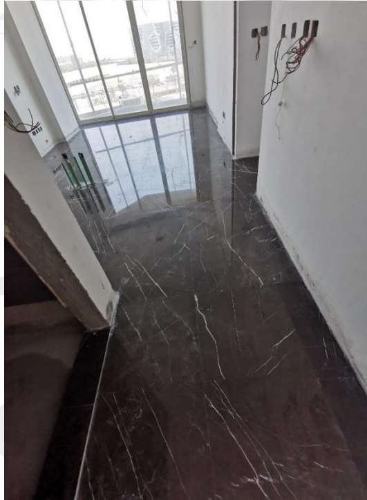
Marble Flooring works at Typical Floors
