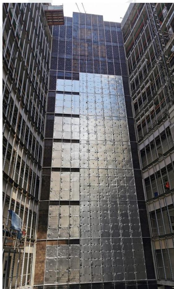
Installation of Aluminum Works (Brackets, Mullion, Rockwool ACP Cladding & Glass and Application of Bitumen Paint)
