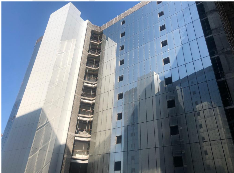
Installation of Aluminum Work (Brakets, Mullion, Rockwool, ACP Cladding and Glass)
