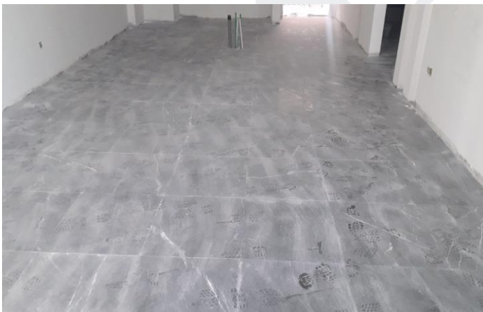
Marble Works at Typical Floors
