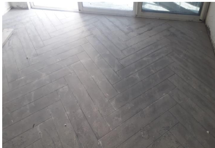
Tile Works at Typical Floors
