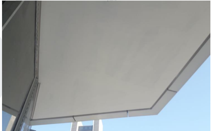
Gypsum Ceiling and Painting Works for Balcony Area at Typical Floors
