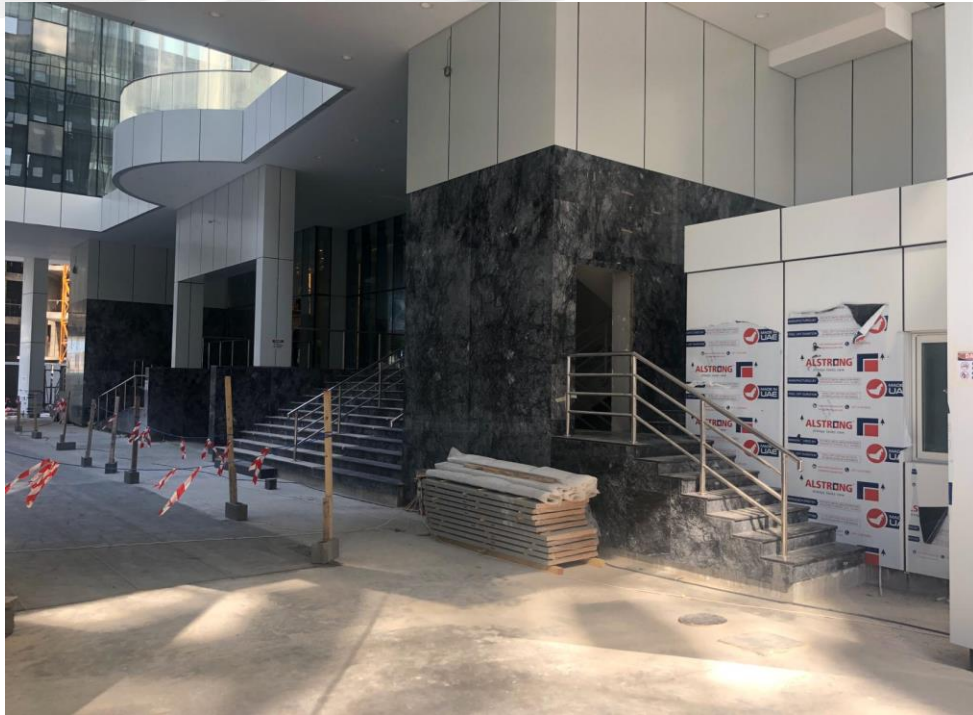
Main Entrance (Ground Floor)
