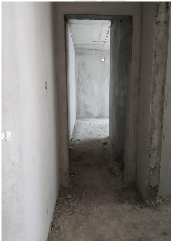
Plastering Works at Typical Floors
