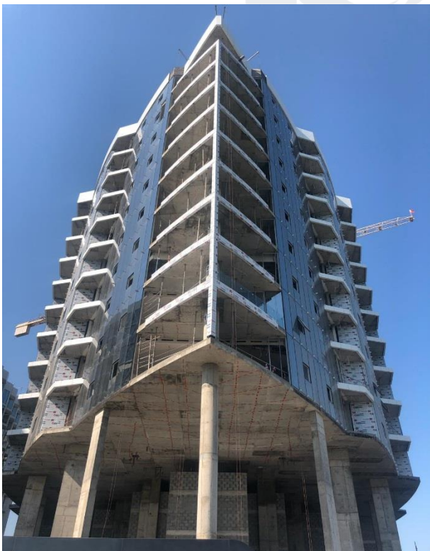
Installation of Aluminum Works (Brackets, Mullion, Rockwool, ACP Cladding and Glass)
