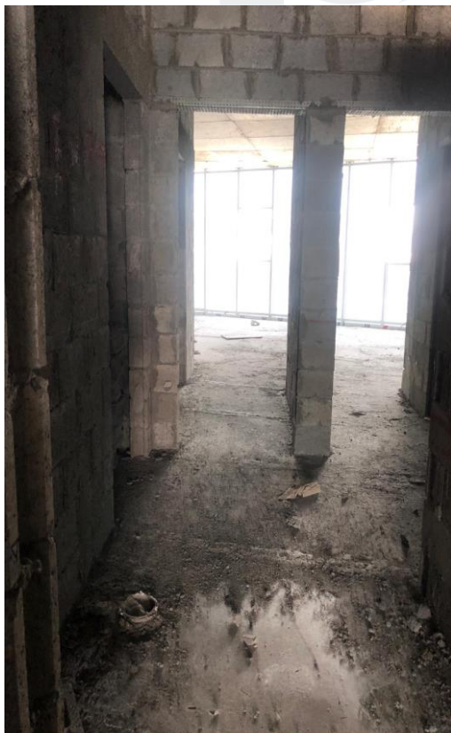
Block Works Lintel Works at Typical Floors
