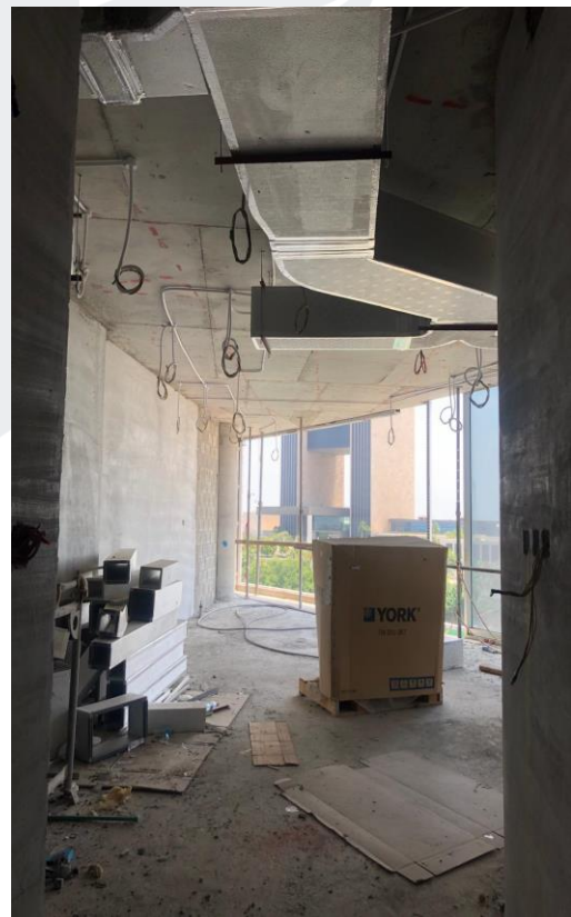
MEP Works at Typical Floors
