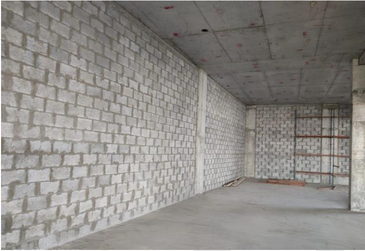
6 th Floor Car Parking Block Work
