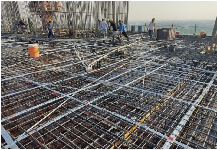
13 th Floor – Slab Reinforcement Works
