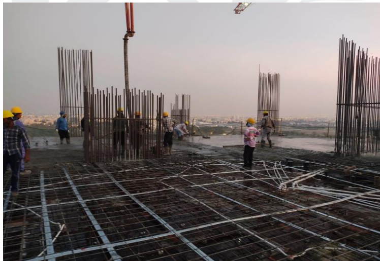
11 th Floor – Shear Wall Concrete Work
