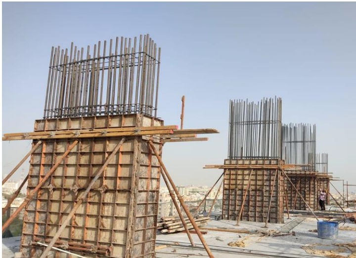
12 th Floor Column Form Work
