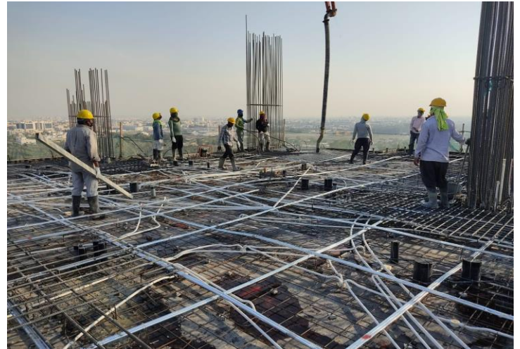
13 th Floor – Slab Reinforcement Works
