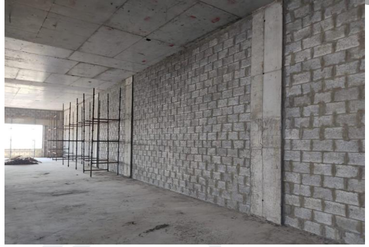
6 th Floor Car Parking Block Work
