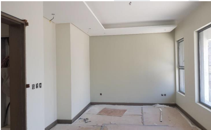
Internal paint application in progress
