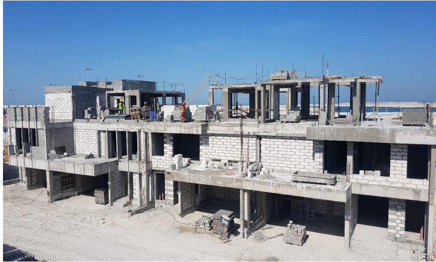
Structural works in progress
