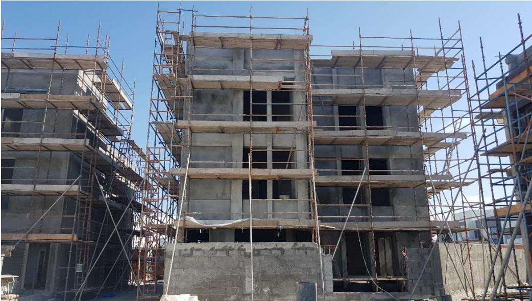
External plastering works in progress
