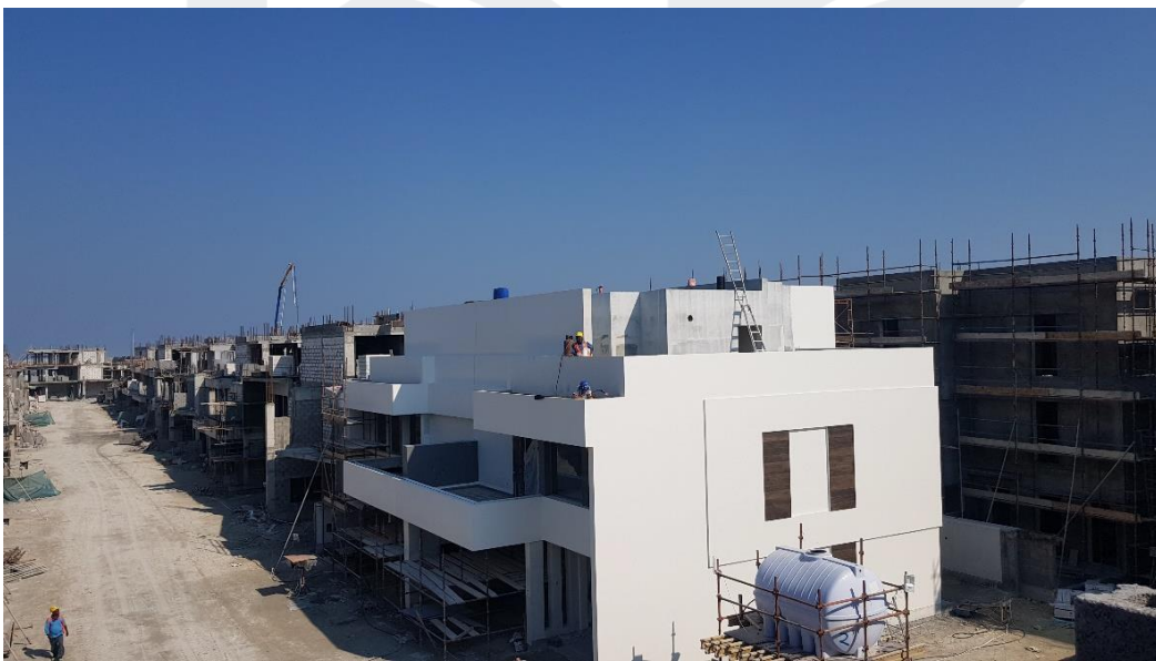
External pain application in progress
