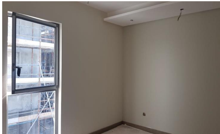
Aluminum Works in progress
