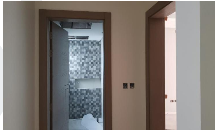
Internal Door installation in progress
