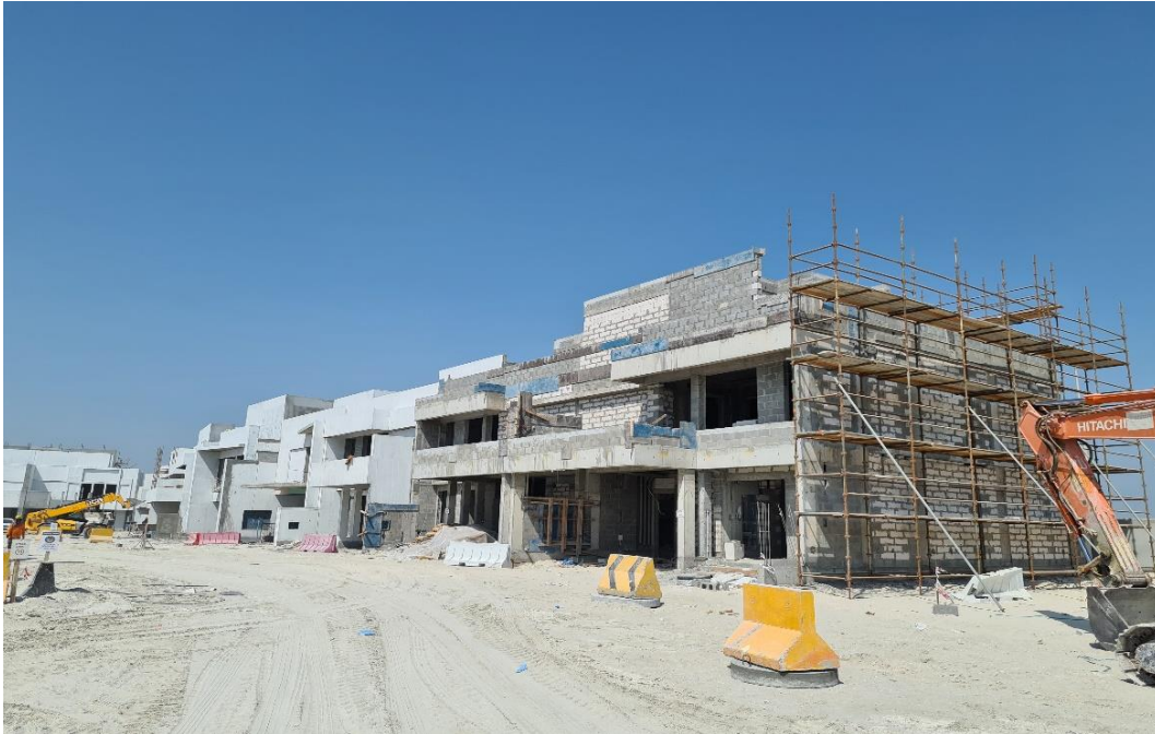
External Plastering preparation works in progress
