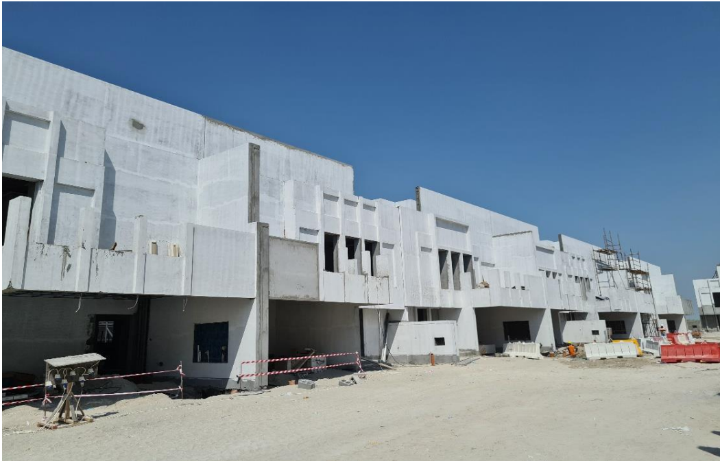
External Finishing works in progress
