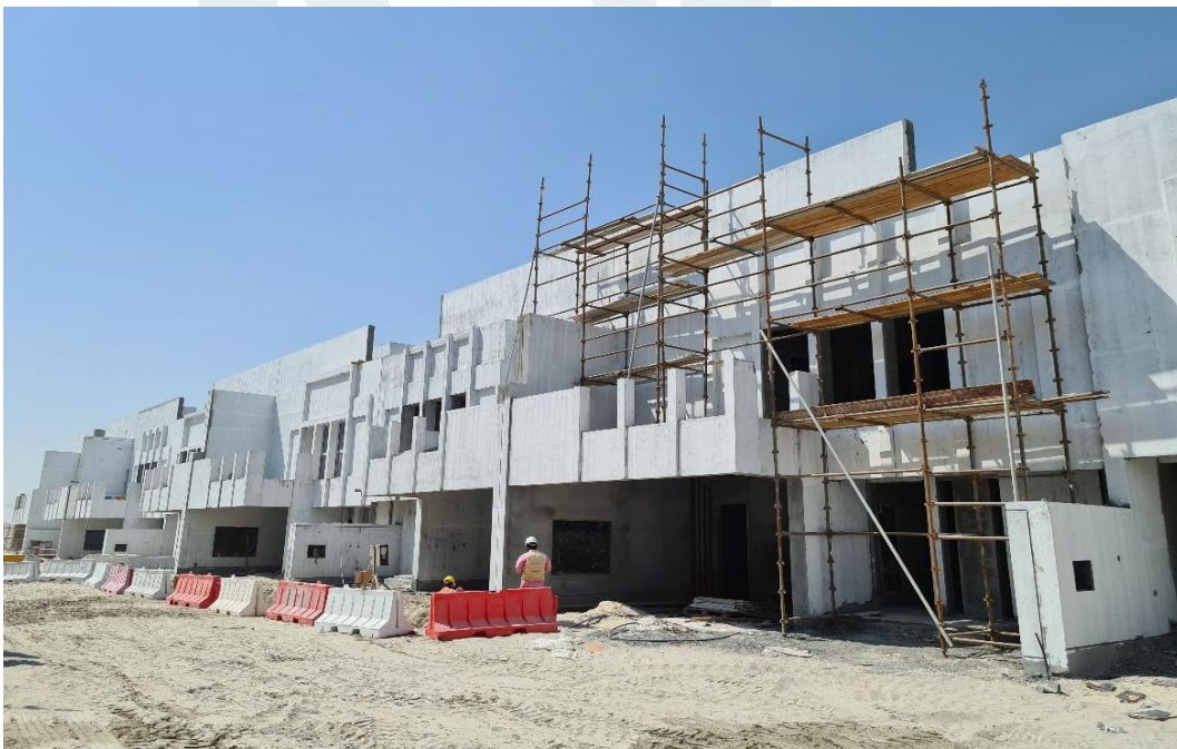
External Painting works in progress
