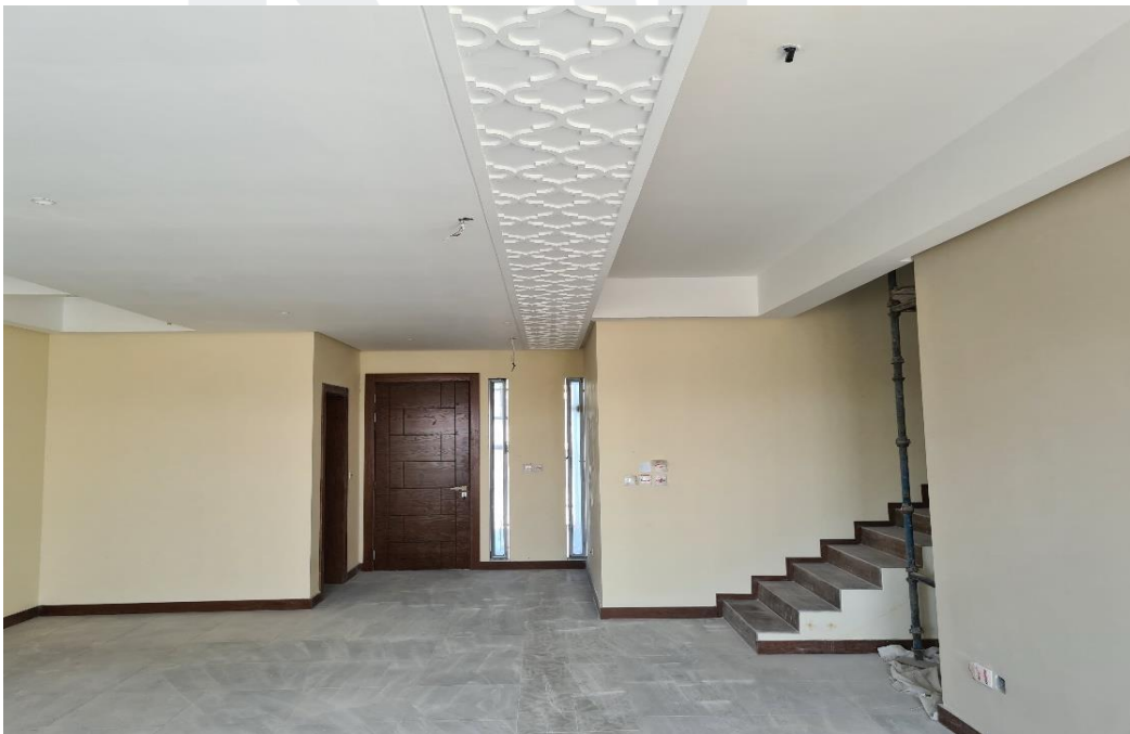
Internal Paint application in progress
