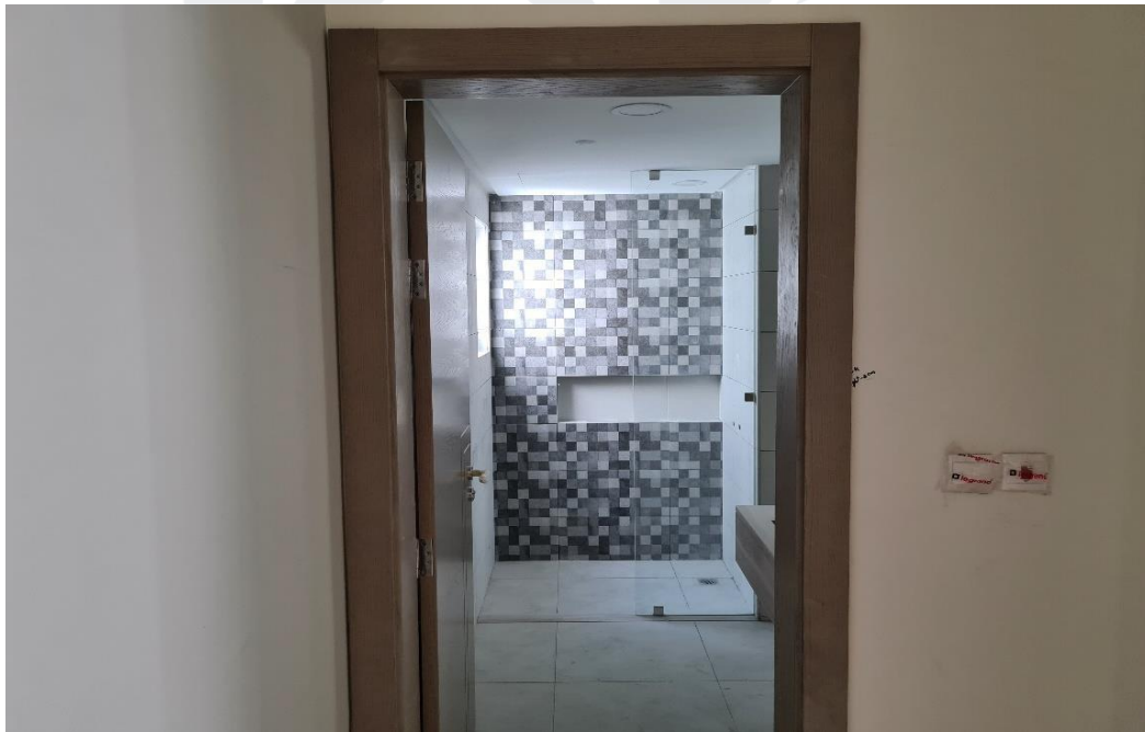
Toilet Shower partition installation in progress
