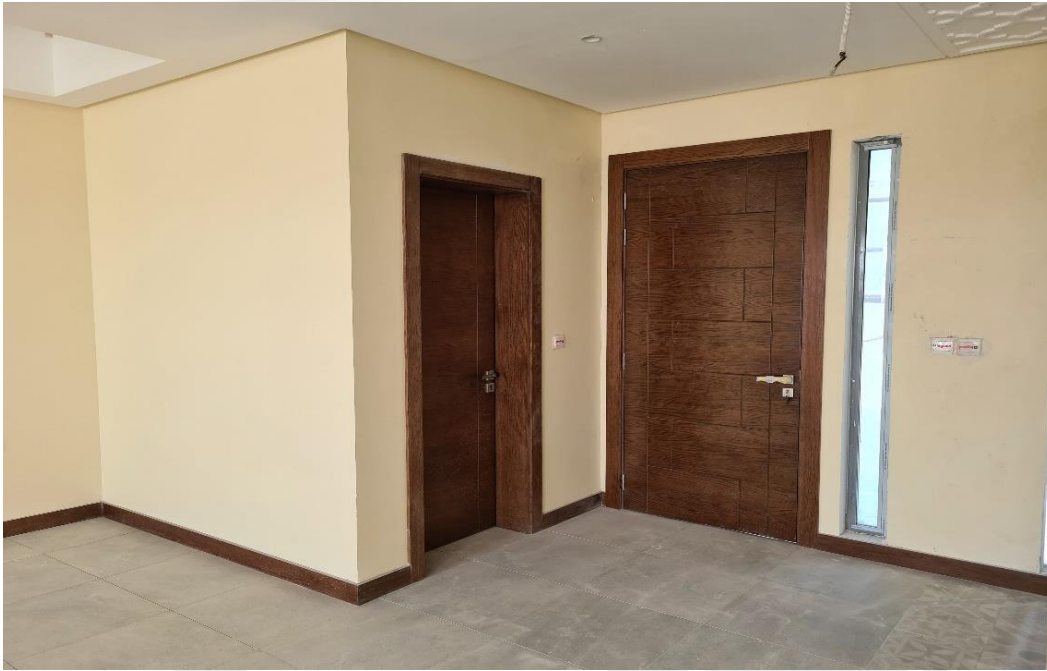
Wooden Doors and Skirting installation in progress
