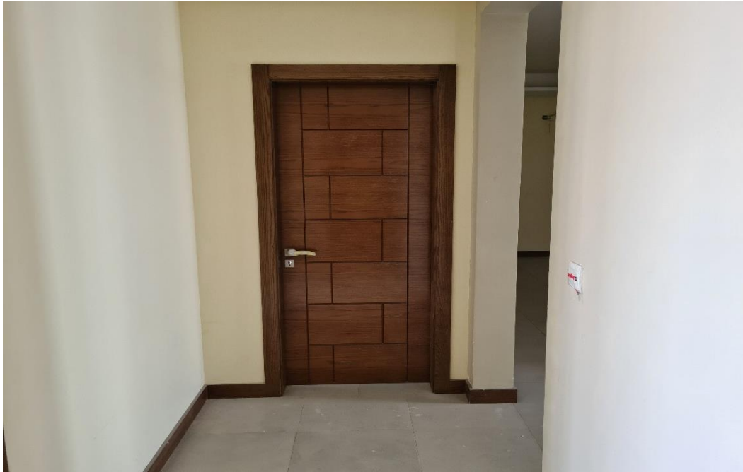
Wooden Doors and Skirting installation in progress
