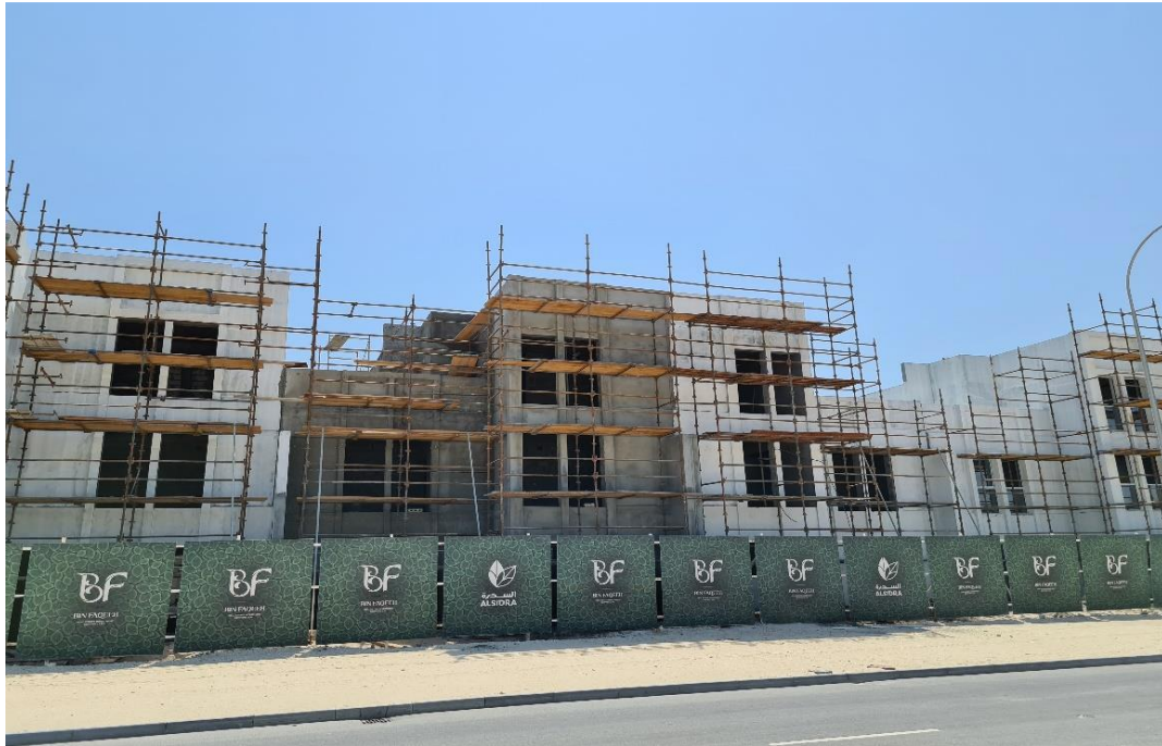
External Plastering works in progress
