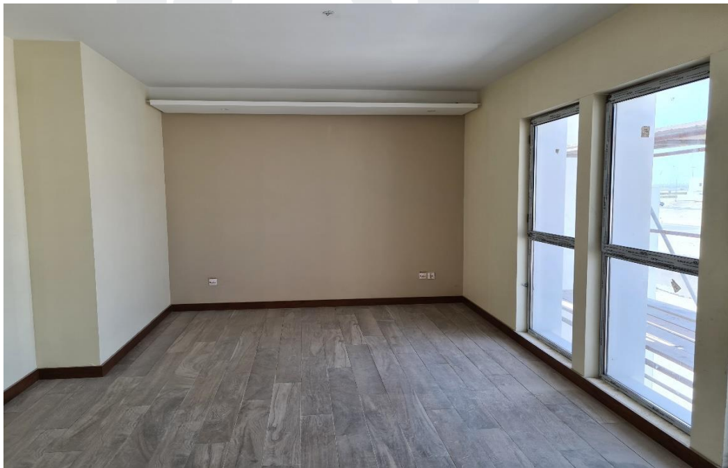
Aluminum Windows installation in progress
