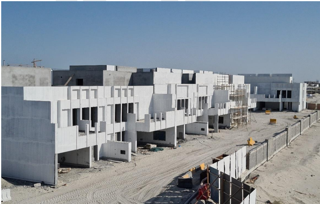
External Painting works in progress
