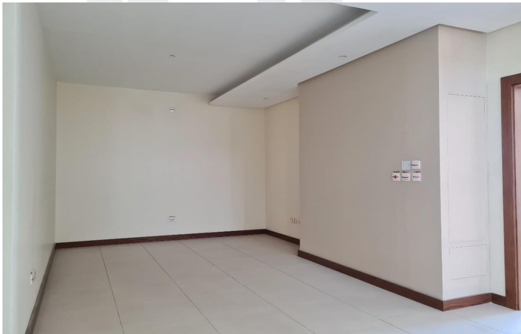
Internal Paint application in progress
