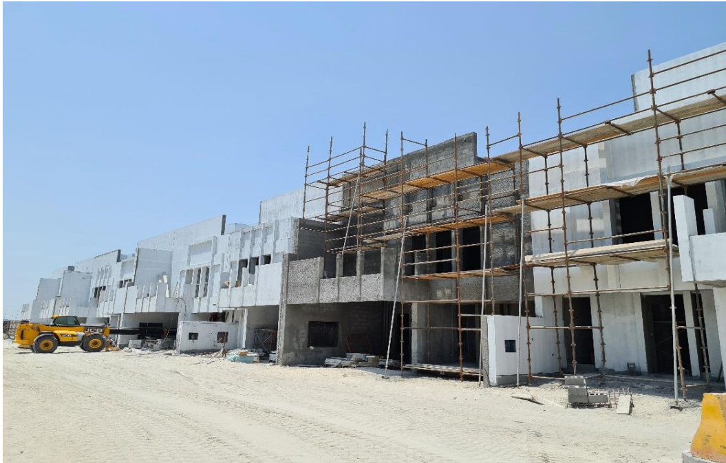
External Plastering Prep works in progress
