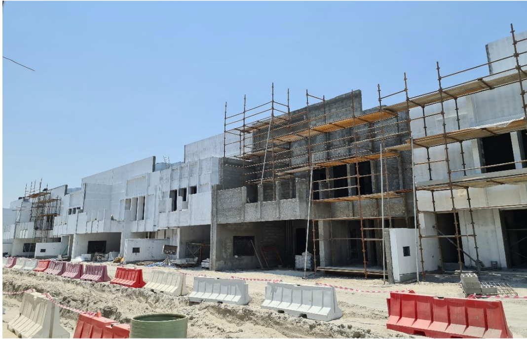
External Plastering works in progress
