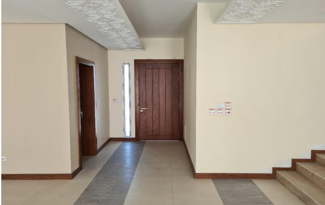
Wooden Doors and Skirting installation in progress
