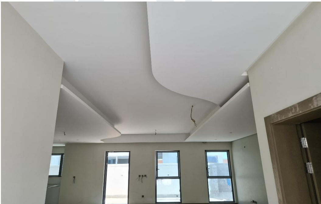
Aluminum Windows installation in progress
