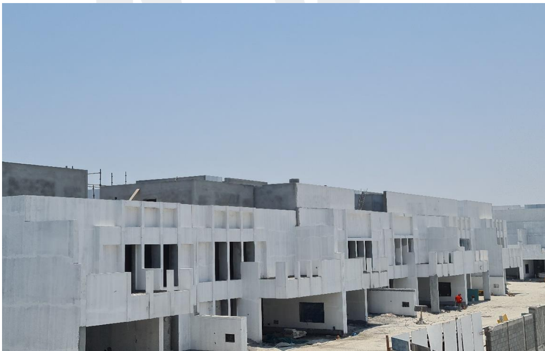
External Painting works in progress
