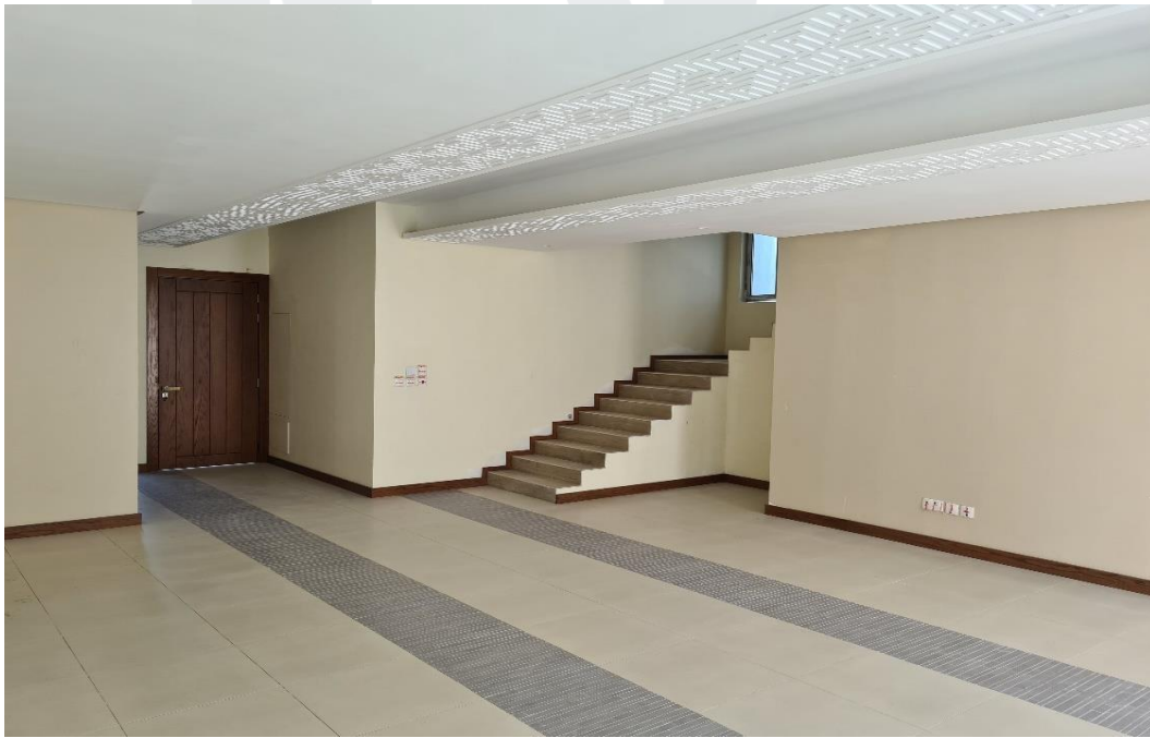
Internal Paint application in progress
