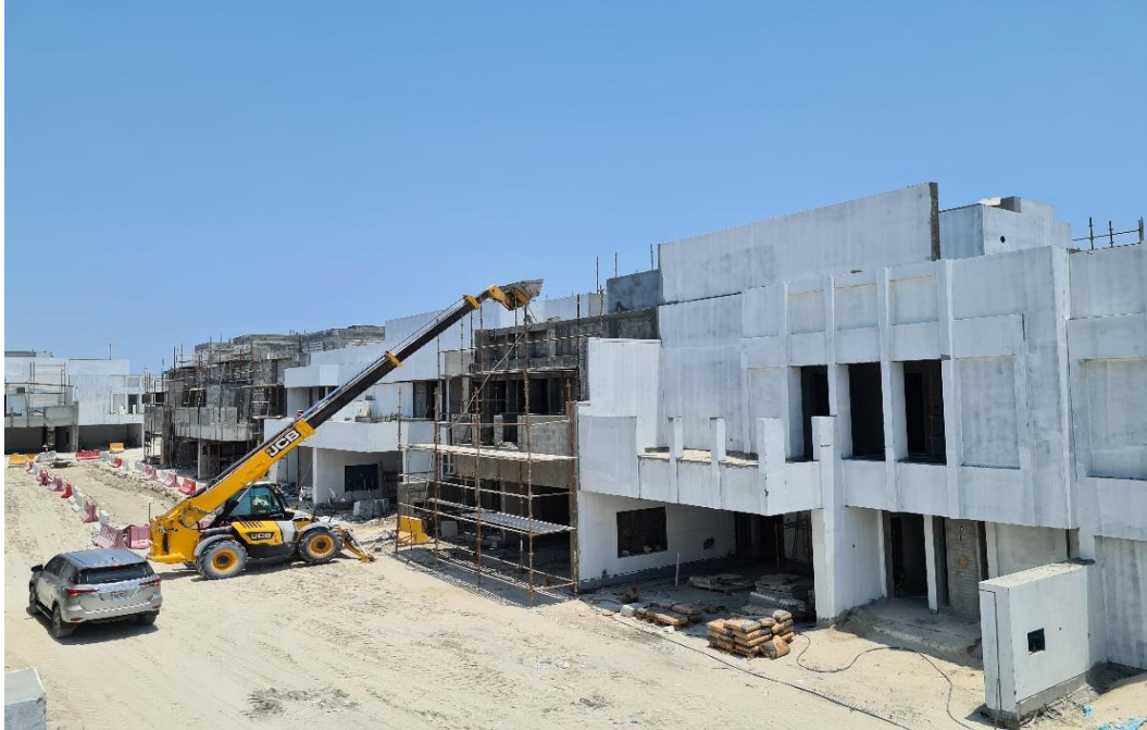
External Plastering works in progress
