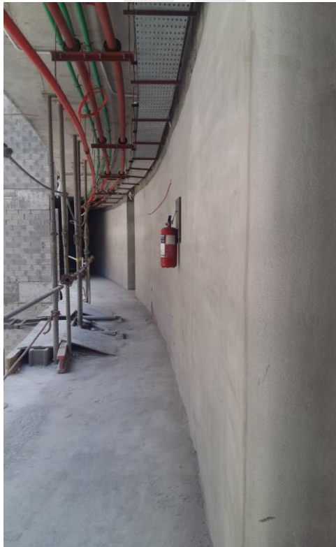
Plastering Works and Installation of MEP Services Works at Typical Floors
