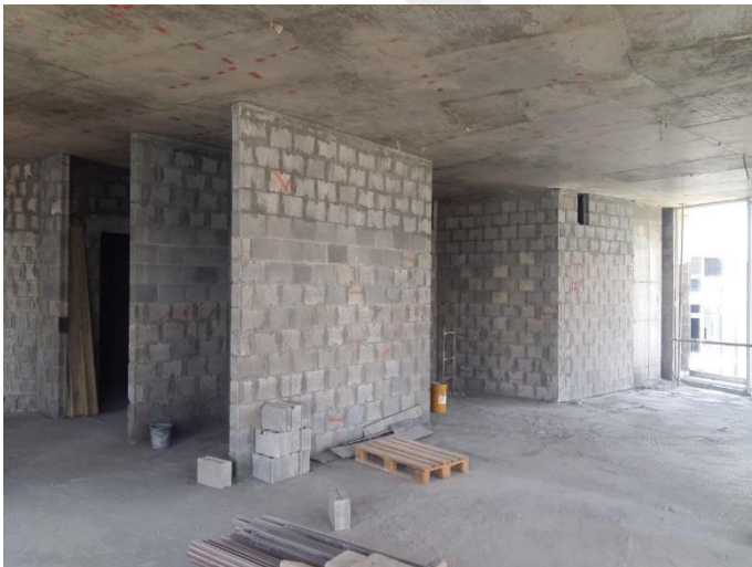
Block Works at Typical Floors
