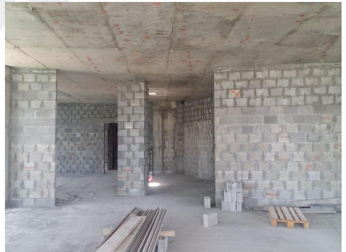
Block Works at Typical Floors
