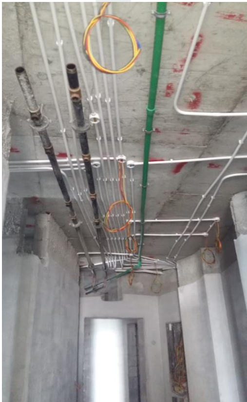
Installation of MEP Services at Typical Floors
