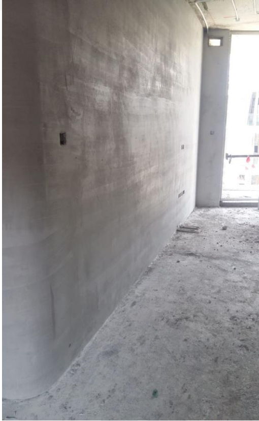
Plastering Works for Walls at Typical Floors
