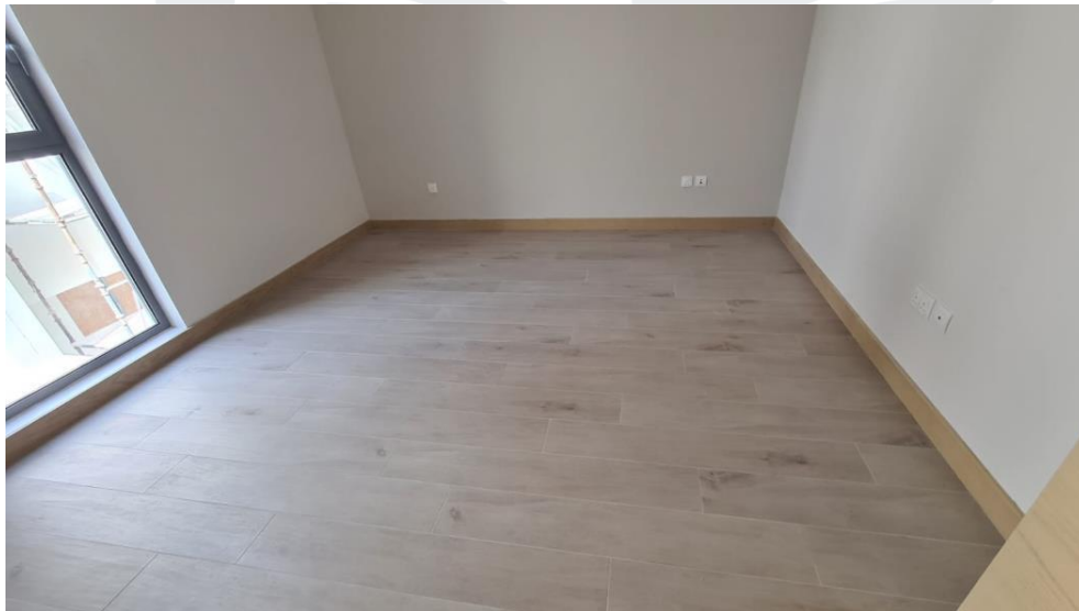
Floor Tile Works Final Finishing in Progress
