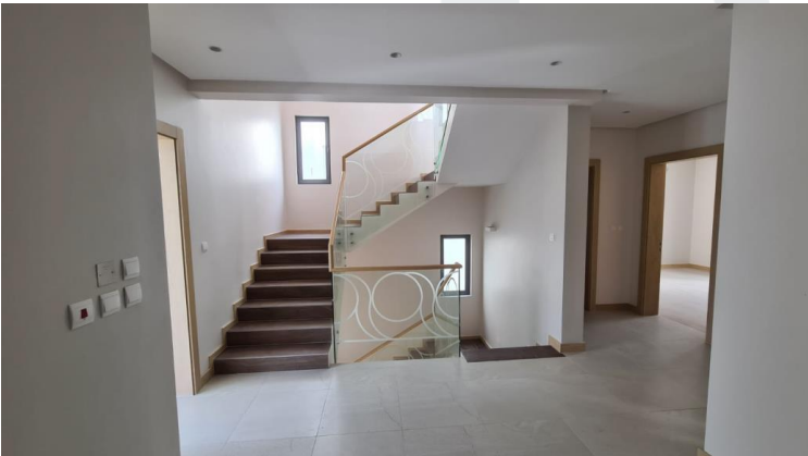
Staircase Handrail Installation in Progress
