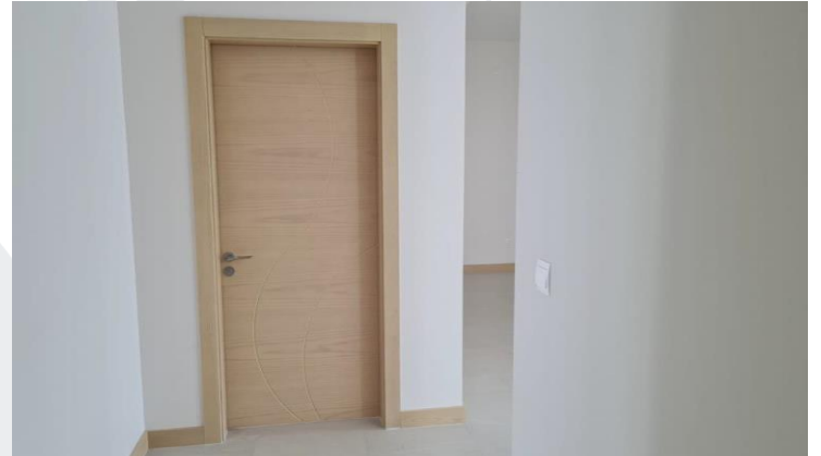
Internal Door Installation in Progress
