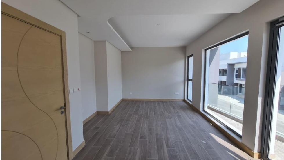
Internal Painting in Progress
