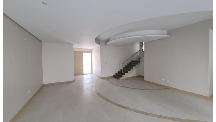
Internal Finishing Works in Progress
