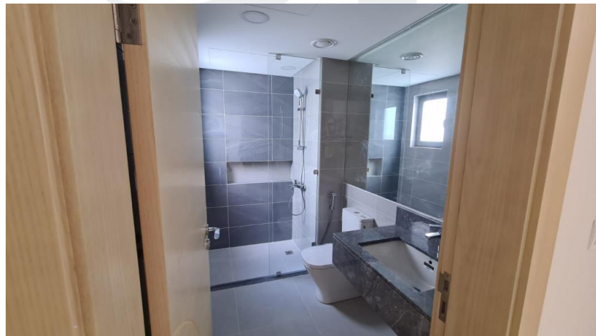
Villa Shower Partition Installation in Progress
