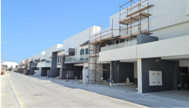
External Painting Works in Progress
