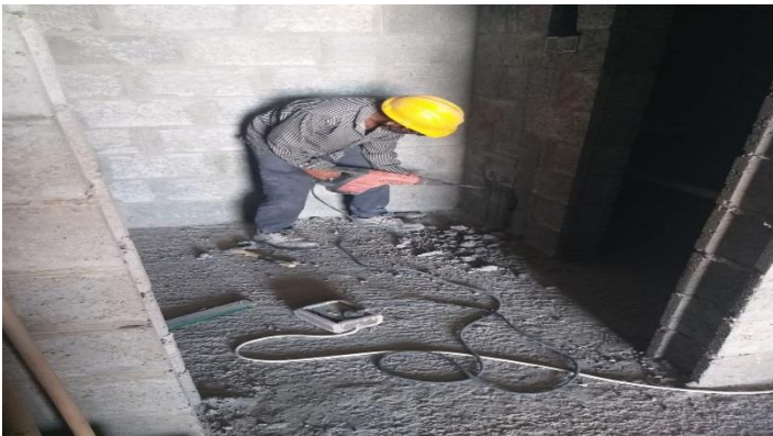
Cutting and Chasing Works
