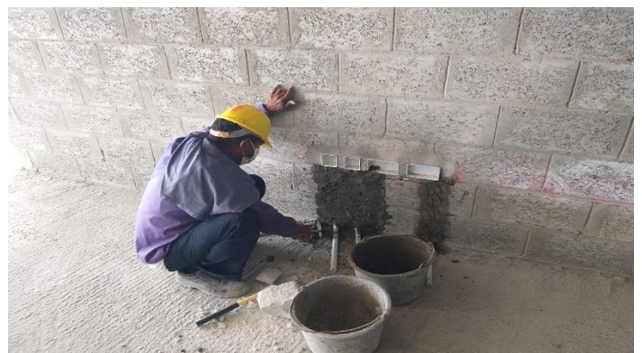
Cutting and Chasing Works
