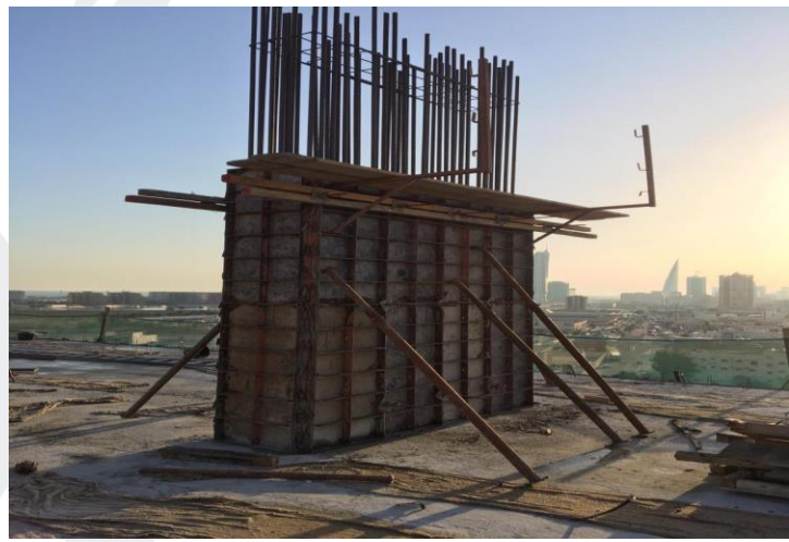
11 th Floor – Column Shuttering Work
