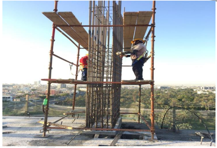
11 th Floor – Column Reinforcement Works
