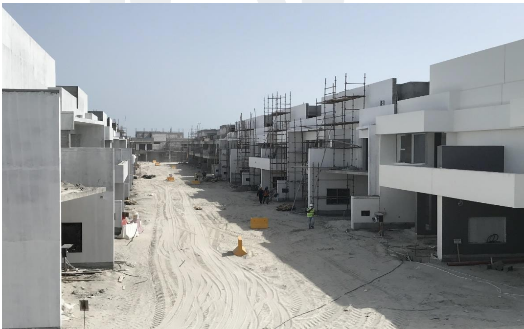
External Painting works in progress
