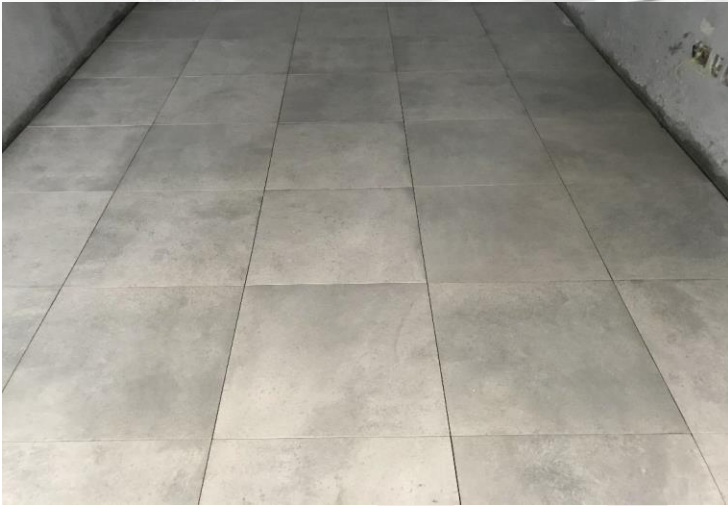
Floor Tile Fixing in progress
