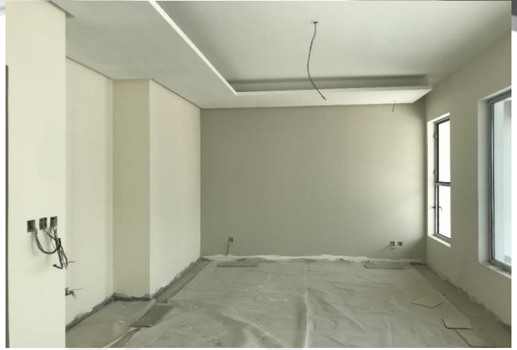
Ceiling works in progress.
