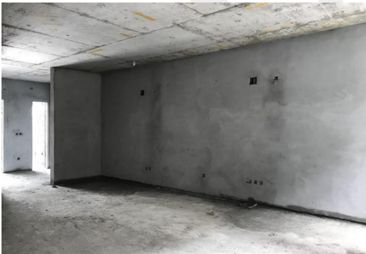
Internal Plastering works in progress
