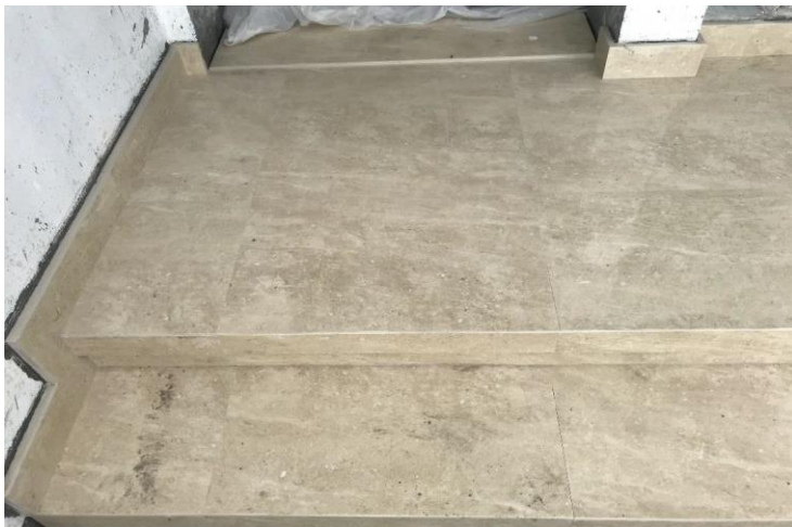
Entrance Floor Tile Installation in progress
