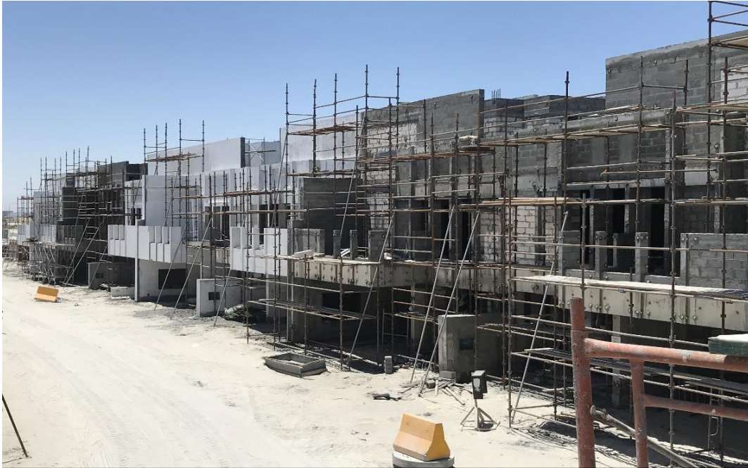
Plastering Preparation works in progress
