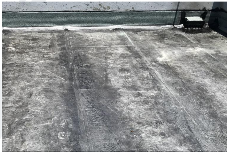
Roof waterproofing works in progress
