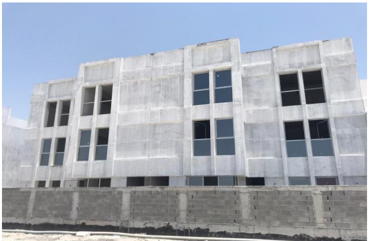
Aluminum Installation Works in progress
