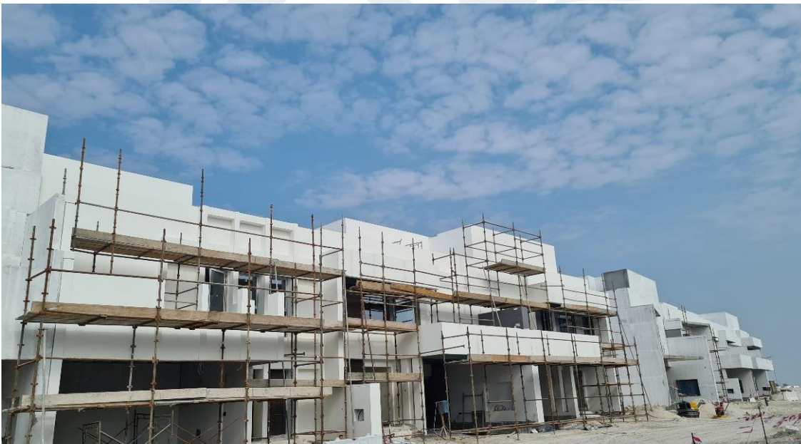
External Painting works in progress
