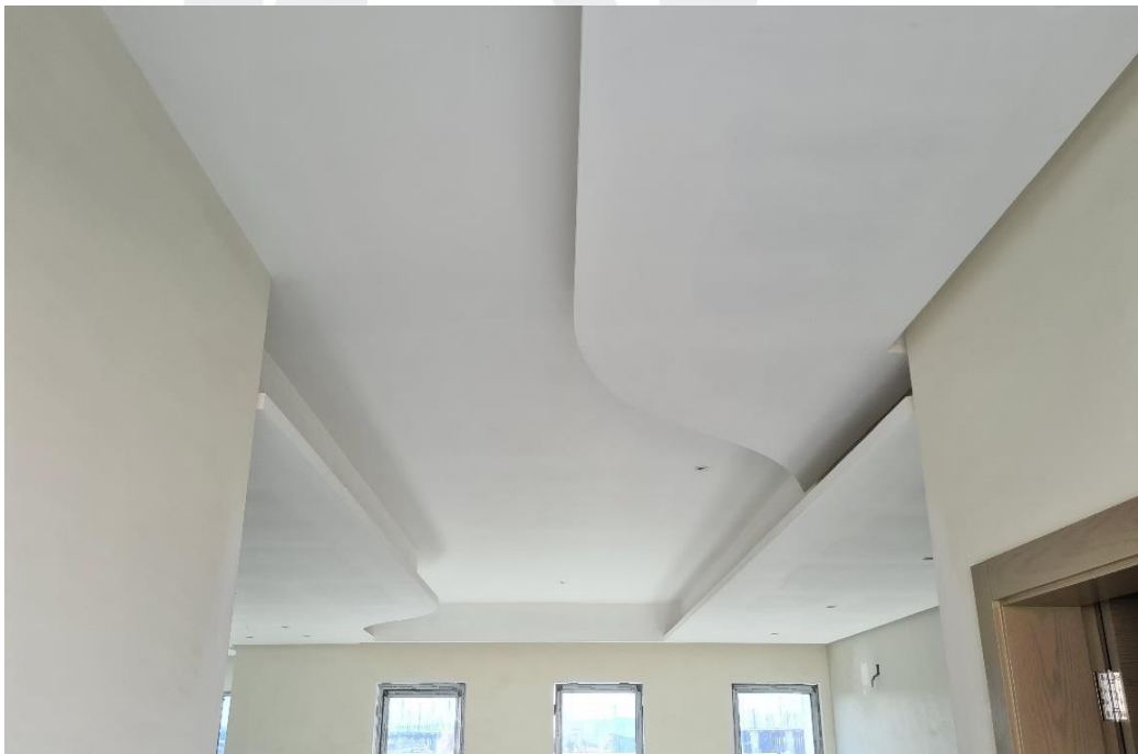
Villas Ceiling works in progress
