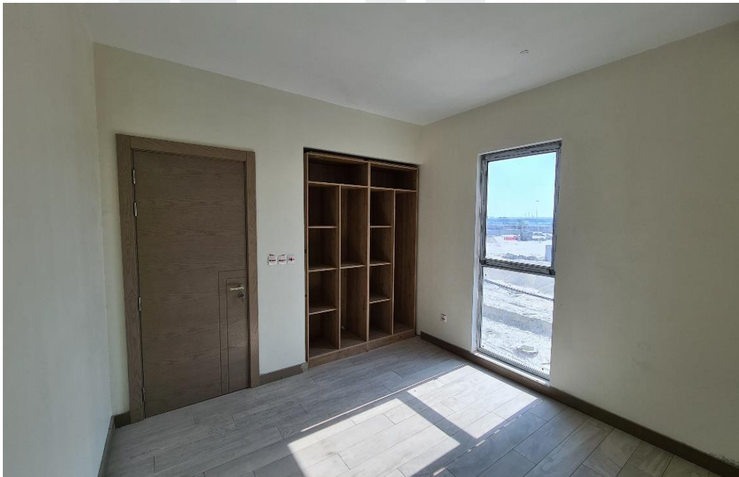
Wardrobe Installation in progress
