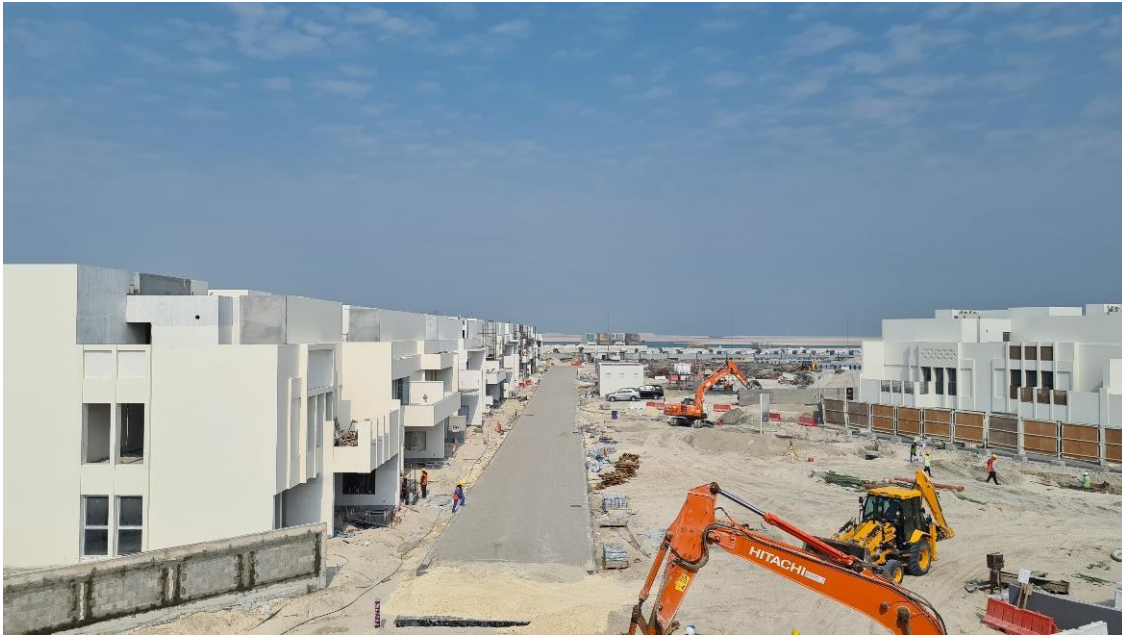
Street View Phase 1A Villas
