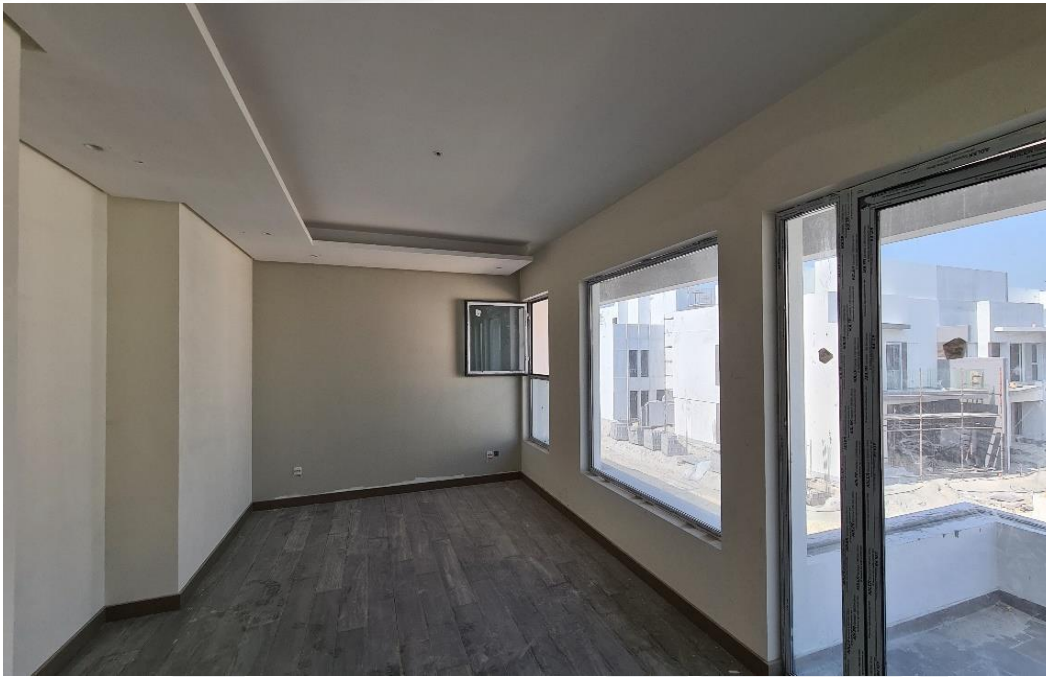
Aluminum Windows installation in progress
