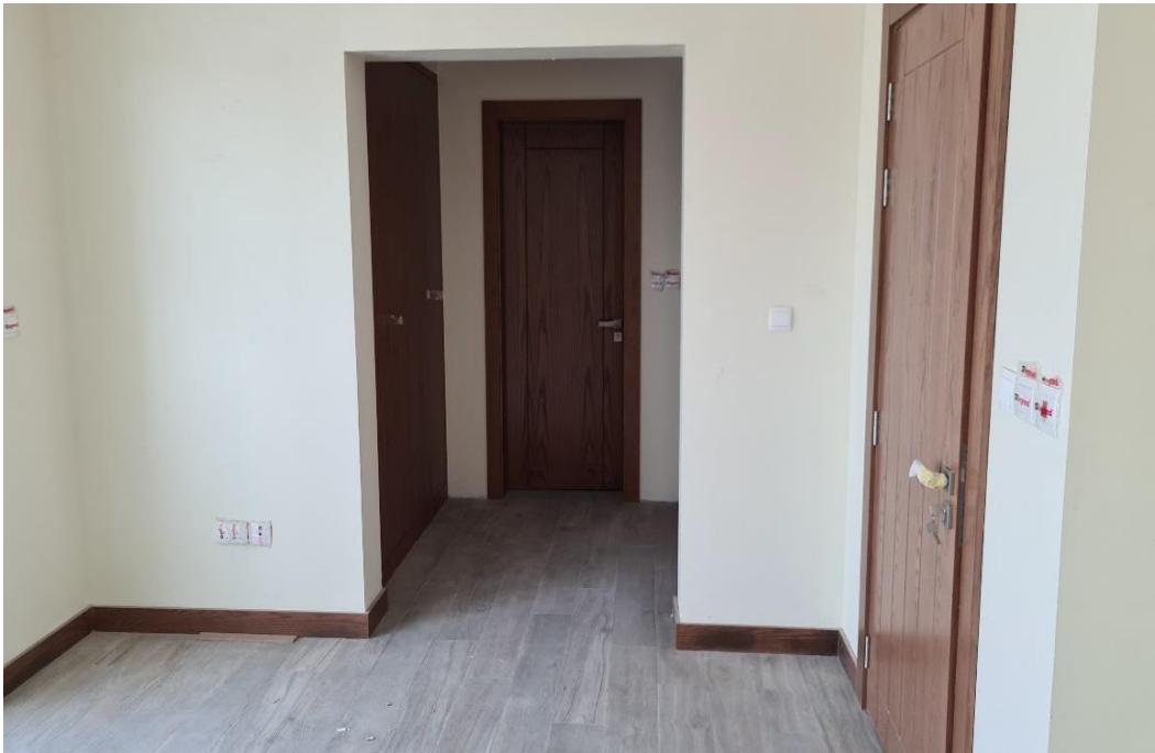
Wooden Doors & Skirting installation in progress
