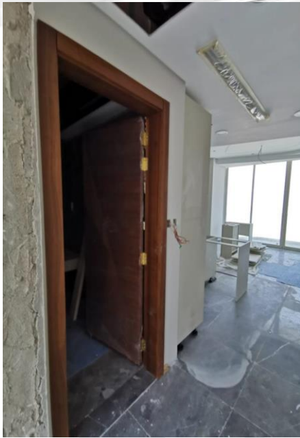
Installation of Doors at Typical Floors
