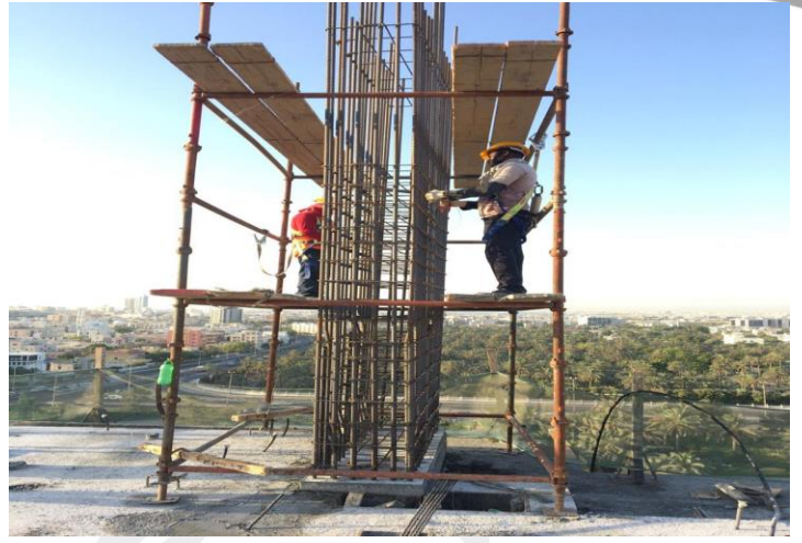
11 th Floor – Column Reinforcement Works
