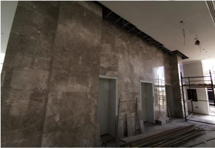
Marble Wall Cladding Works for Lift Lobby Area at Typical Floors
