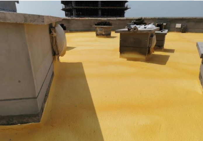
Waterproofing Works at Roof Floor
