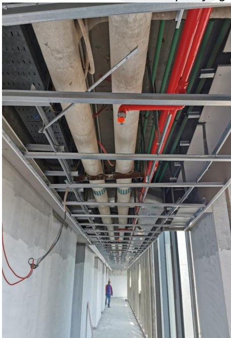
Installation of MEP Services at Typical Floors
