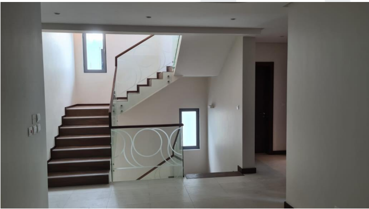
Staircase Handrail Installation in Progress
