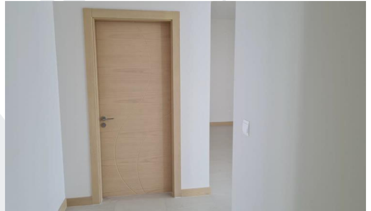
Internal Door Installation in Progress
