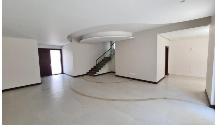
Internal Finishing Works in Progress
