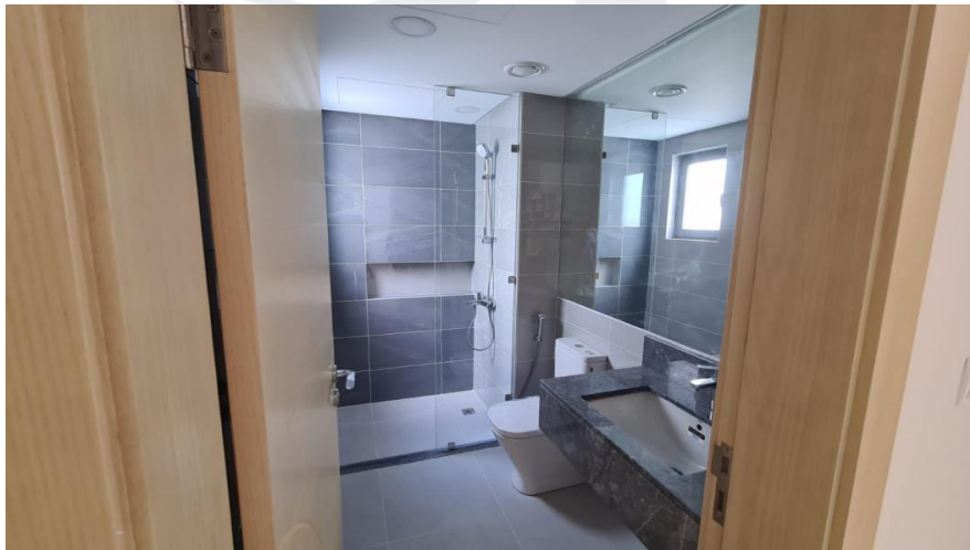
Villa Shower Partition Installation in Progress
