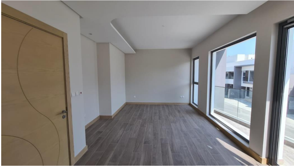
Internal Painting in Progress
