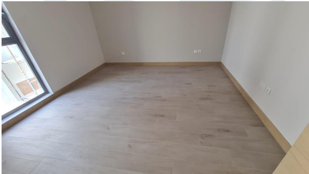
Floor Tile Works Final Finishing in Progress
