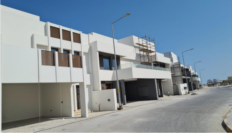
External Painting Works in Progress
