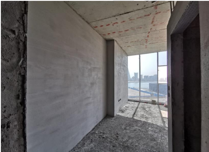
Plastering Works at Typical Floors
