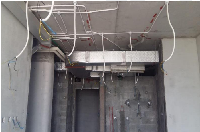
Installation of MEP Services at Typical Floors
