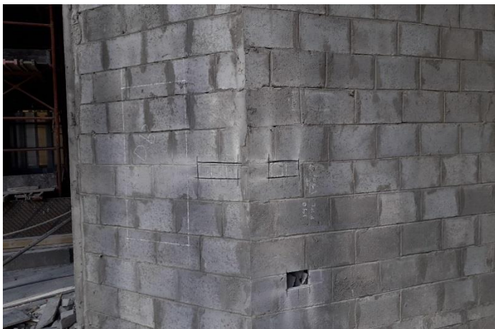
MEP Services Marking Works at Typical Floors
