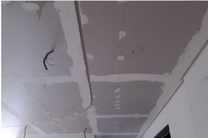
Gypsum Ceiling Painting Works at Typical Floors
