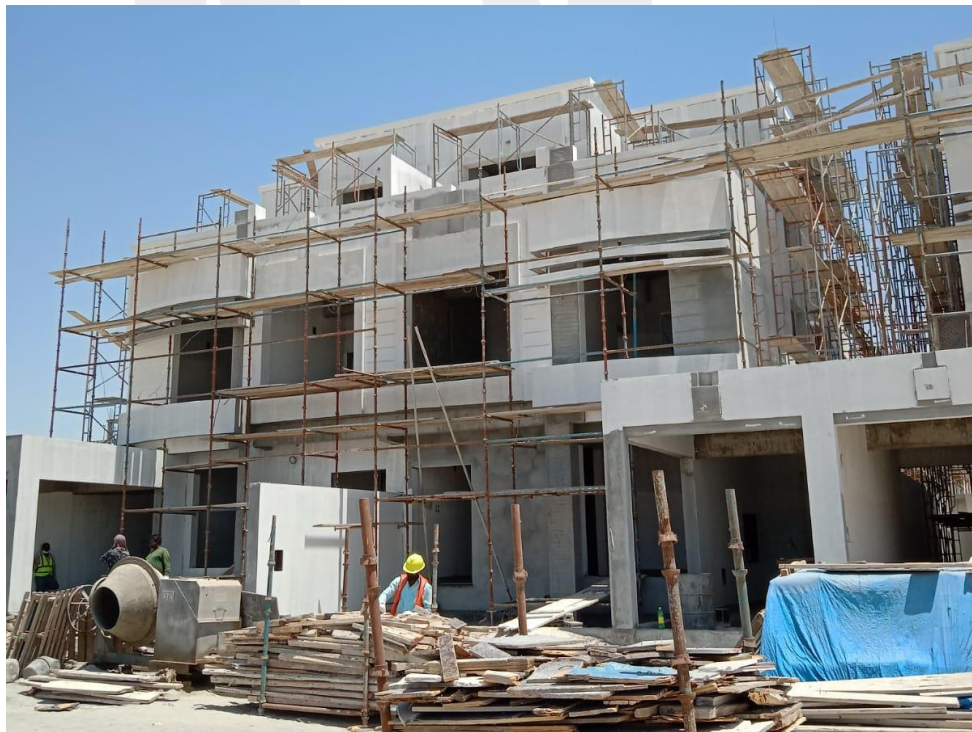
Villa 5 & 6 Overall View
