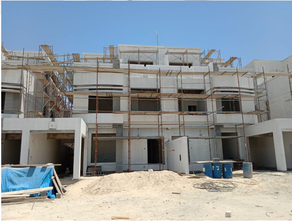
Villa 3 & 4 Overall View
