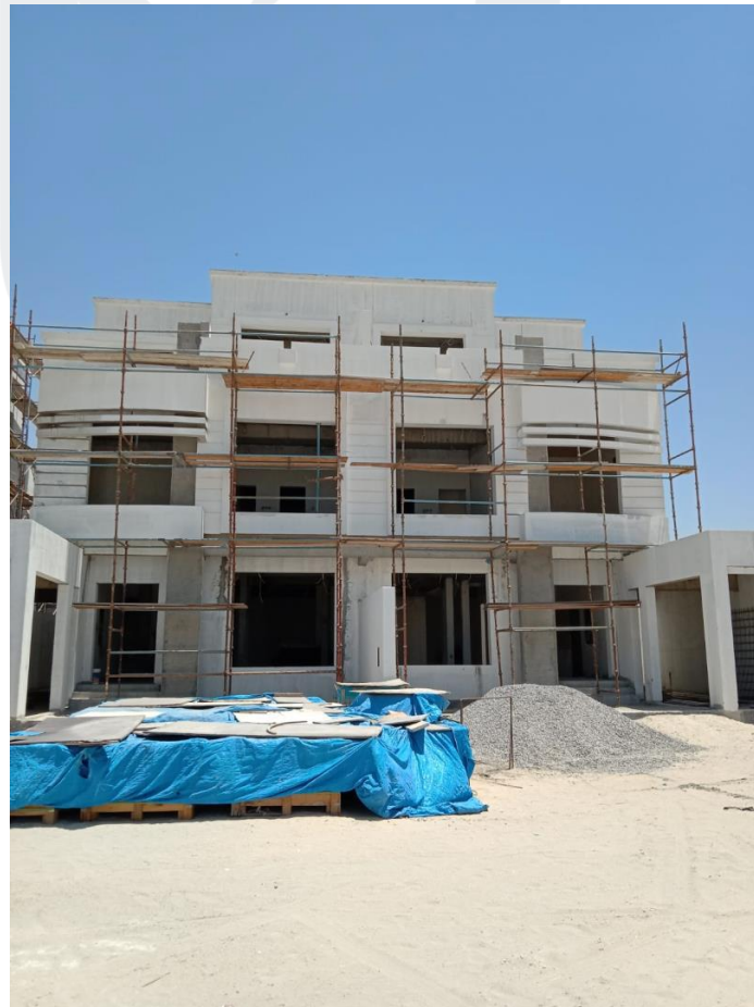
Villa 1 & 2 Overall View
