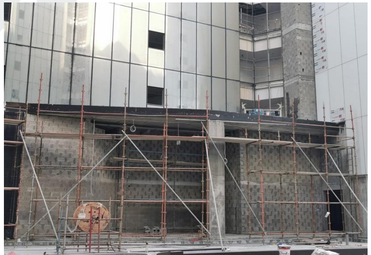
Block Works at Ground Floor
