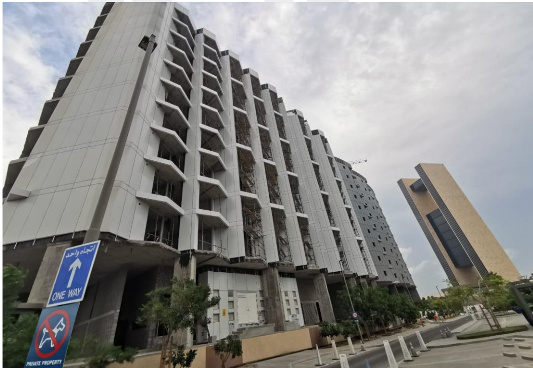
Installation of Aluminum Works (Brakets, Mullion, Rockwool ACP Cladding & Glass and Application of Bitumen Paint)
