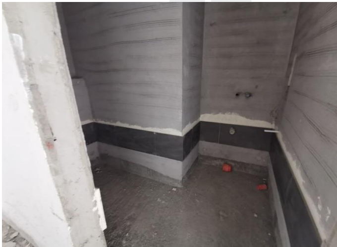
Tile Works for Toilet at Typical Floor
