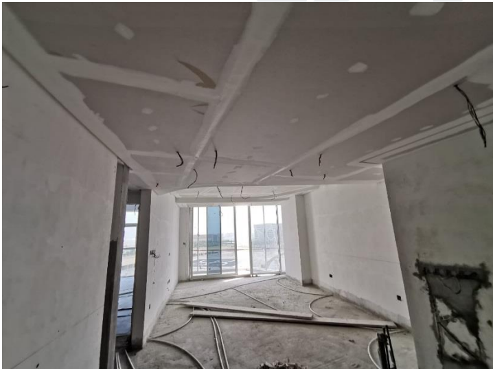
Gypsum Ceiling Works at Typical Floors
